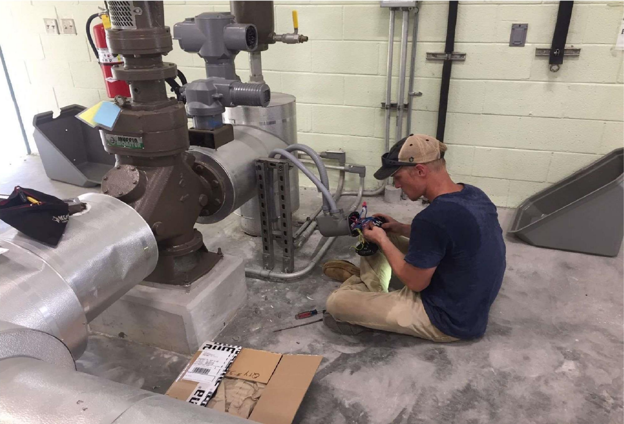
Work on MOVs
