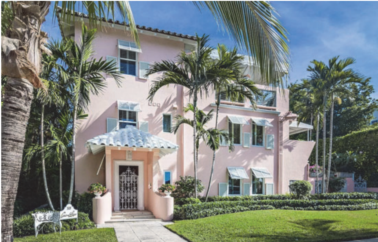
Main (West) Façade
