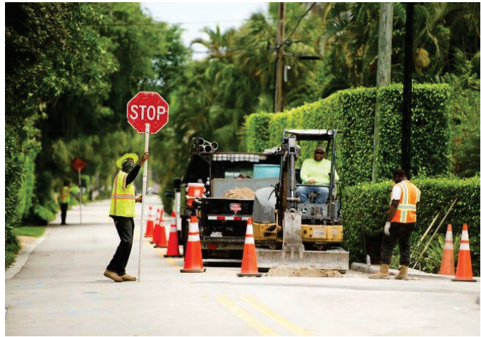
Workers Installing Underground Utilities
