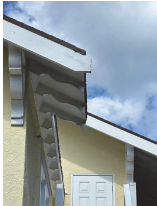
Carved Rafter Tails and Brackets
