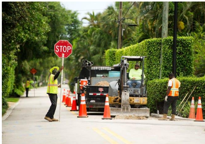
Workers Installing Underground Utilities
