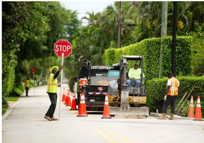
Workers Installing Underground Utilities
