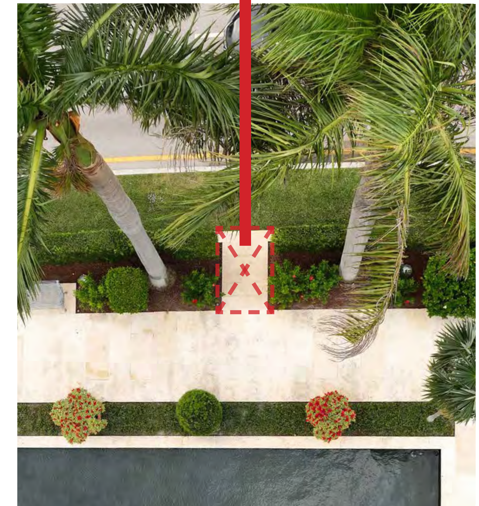
SIDEWALK FACING WEST WITH NO CROSSWALK
