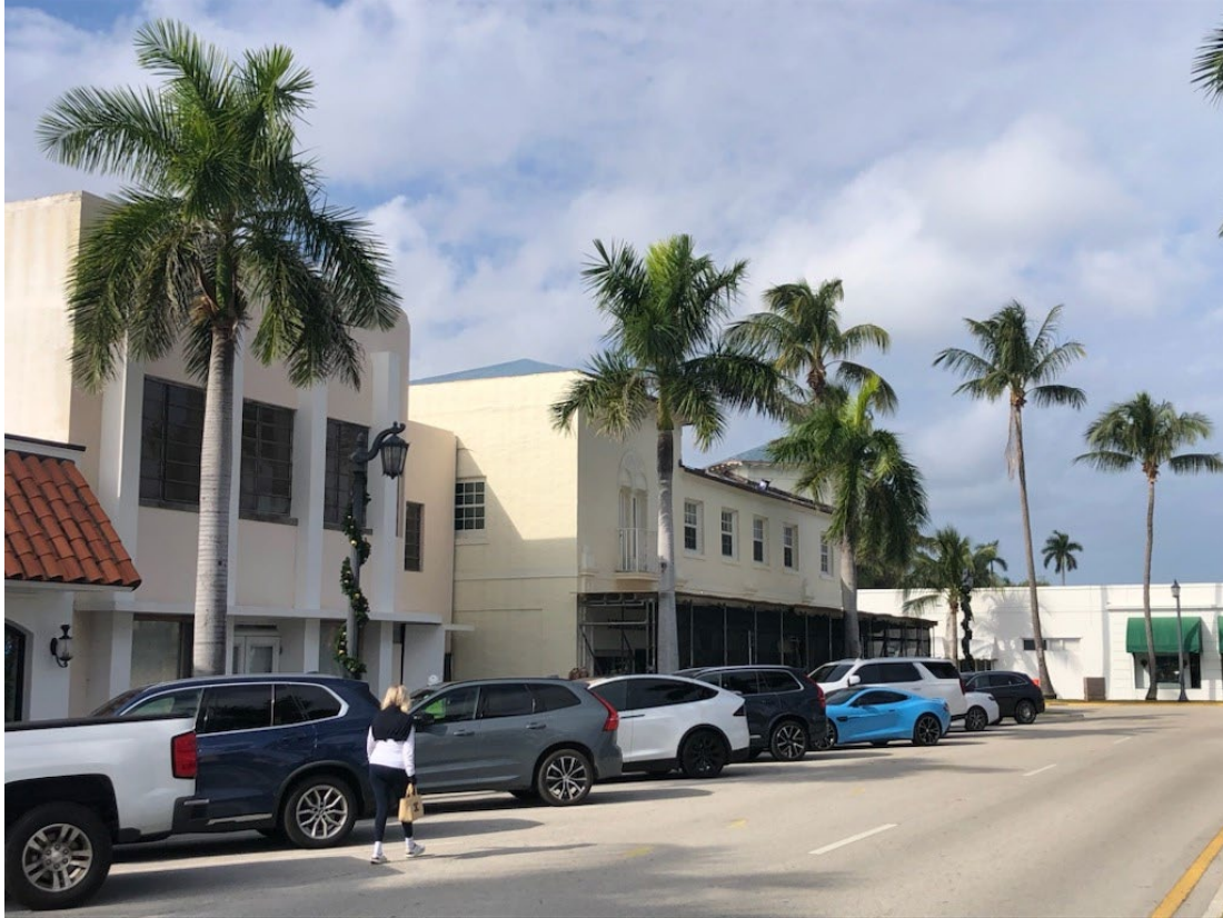
Figure 1- Looking northwest up South County Road at east face of the 870 Brazilian Avenue Building;
