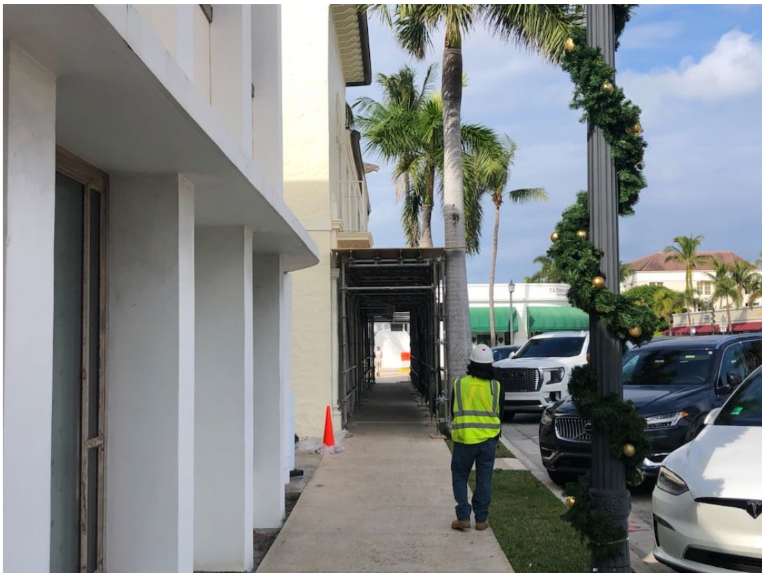
Figure 2- Looking north up the sidewalk of South County Road at the scaffolding protecting pedestrians in front of 870 Brazilian Avenue Building;
