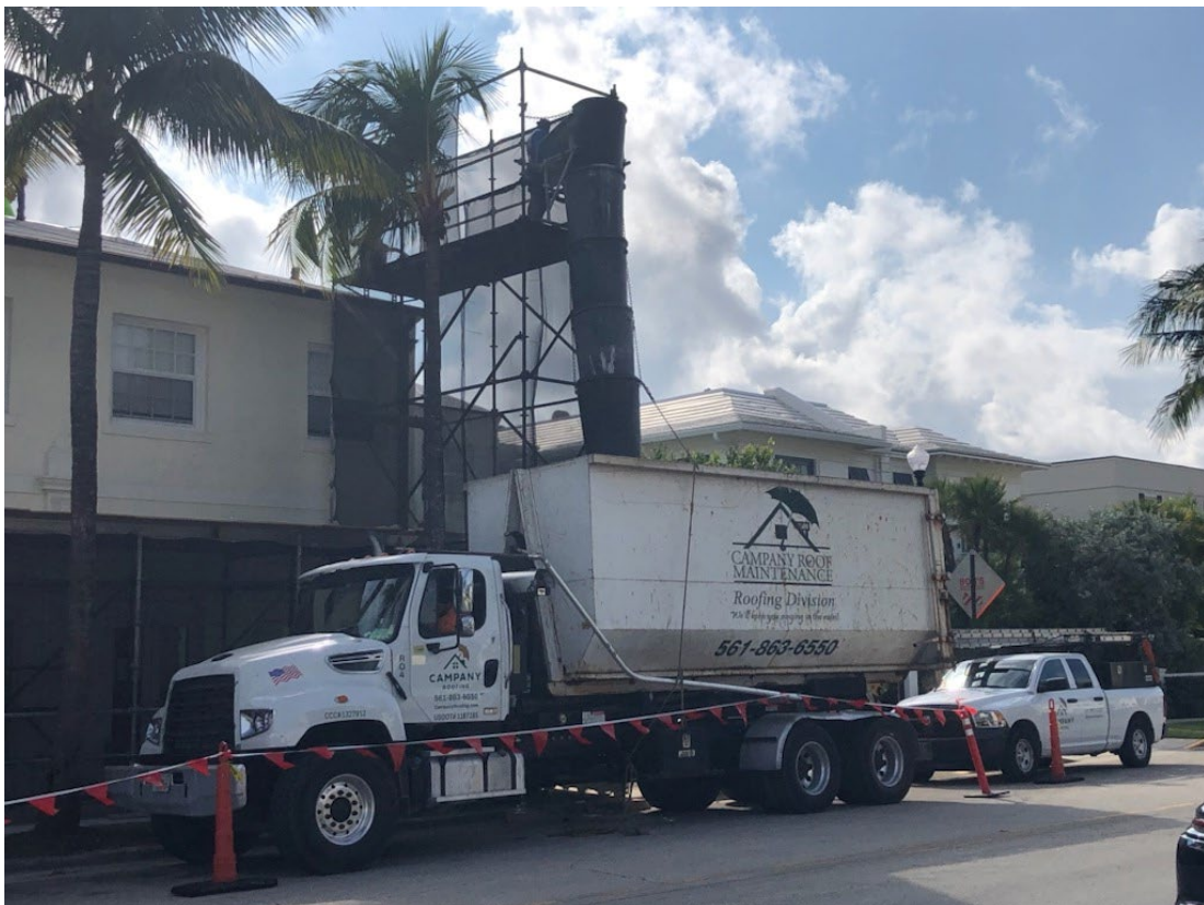
Figure.0.- Looking south from across Brazilian Avenue at the northwest corner of the 870 Brazilian Avenue Building;
