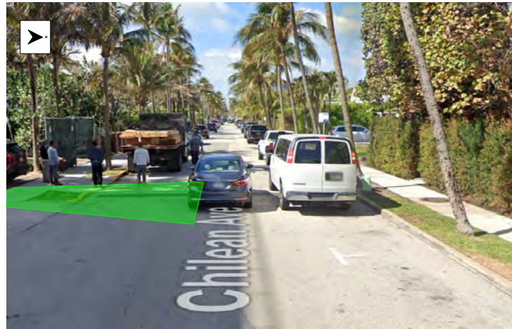
STREET VIEW OF WORK AREA
