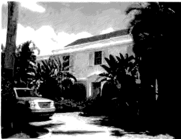
235 Sanford Avenue, Wyeth and King, 1940
