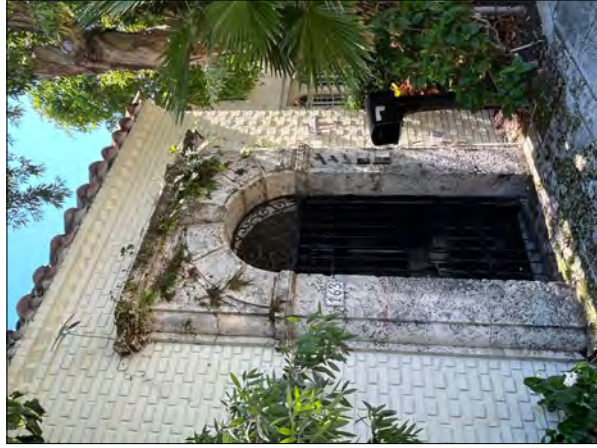
163 SEMINOLE - ENTRANCE GATES
