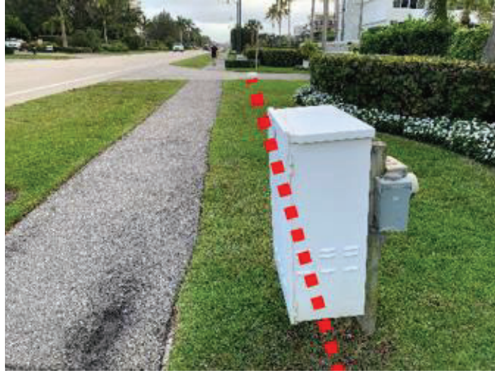
Existing Communications Utility Panel
