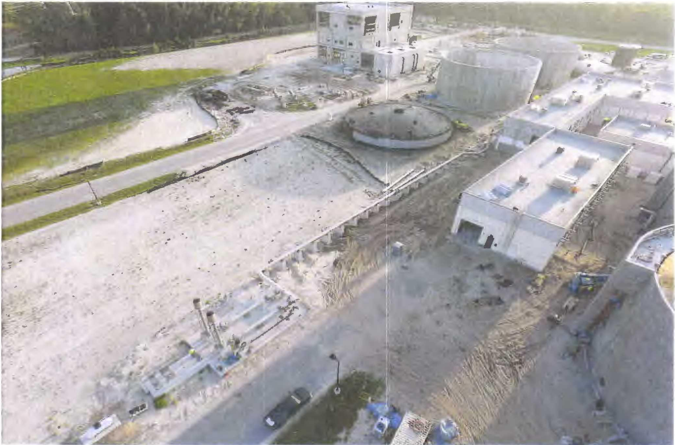
Waste Gas Burners
