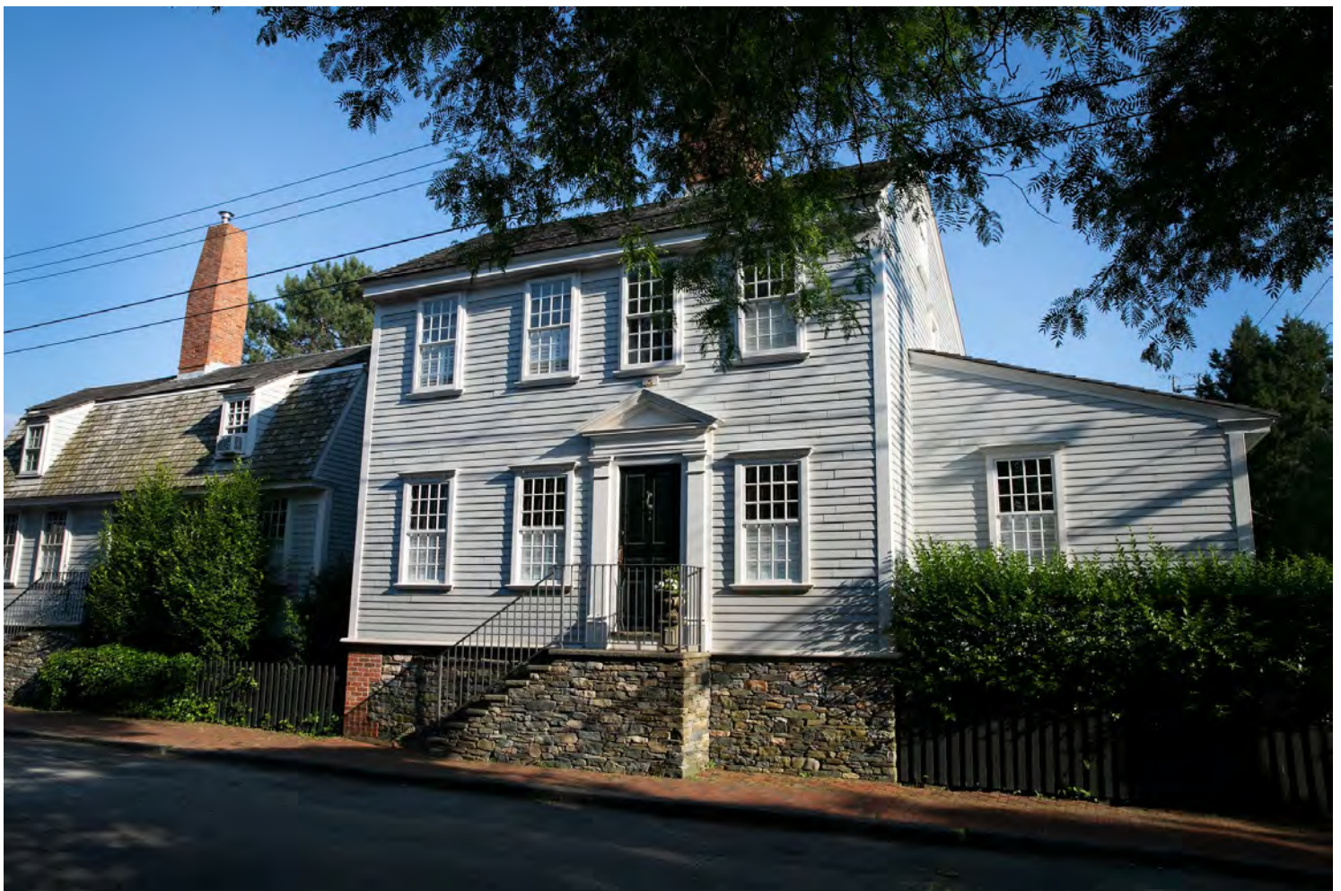
The John Townsend House, which has been elevated for protection from sea level rise. Kayana Szymczak for The New York Times
