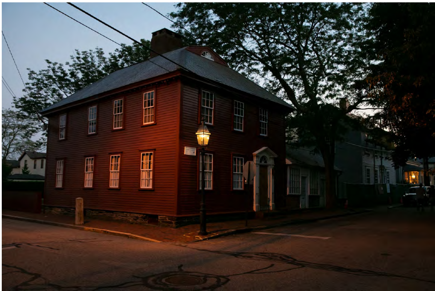
The Christopher Townsend House at 74 Bridge Street. The home has been a test case for architects and engineers searching for ways to rescue Colonial-era buildings from rising seas. Kayana Szymczak for The New York Times
