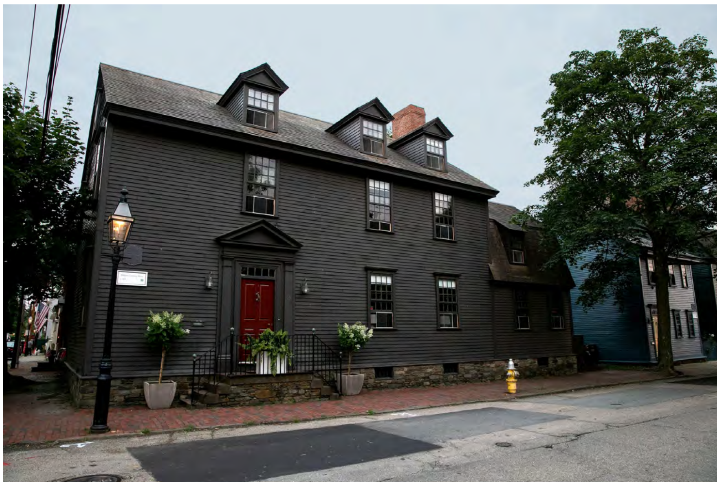
The Jahleel Brenton Counting House, located in The Point. Kayana Szymczak for The New York Times
