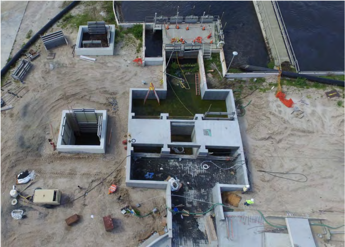
Aeration Basin Influent Structure
