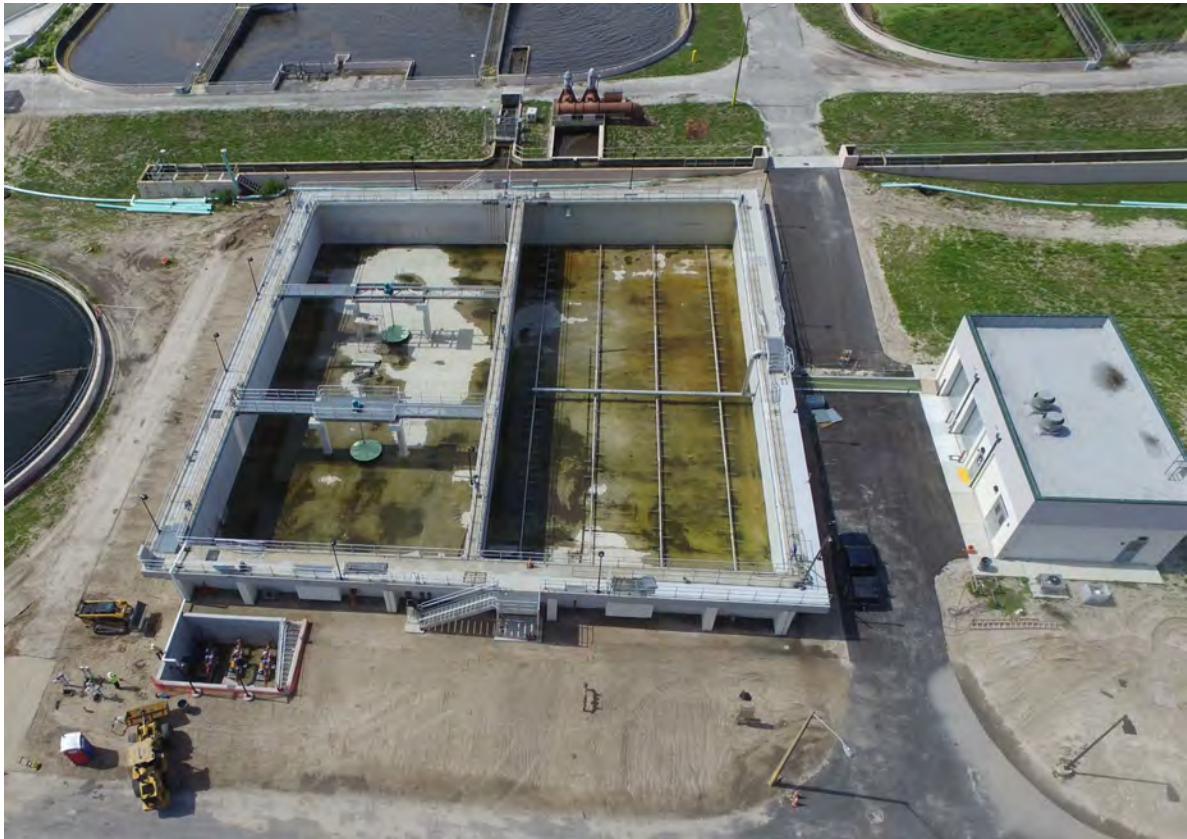
WAS Storage / Centrate EQ / WAS Blower Building
