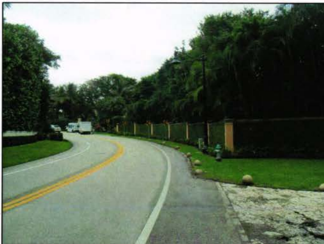
Exhibit 3: Existing Signage at Reverse Curve, Looking Southeast on Southbound SR A1A
