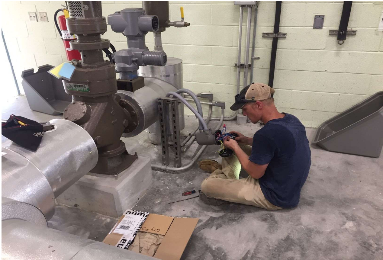
Work on MOVs
