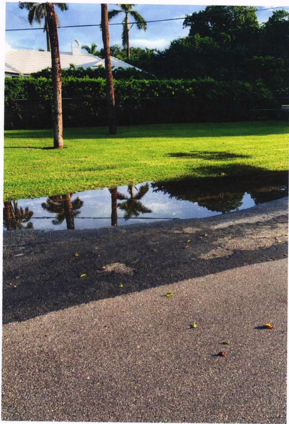
EMERALD - BEFORE NEW DRAINAGE
