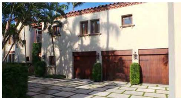
East Façade of Garage Apartment
