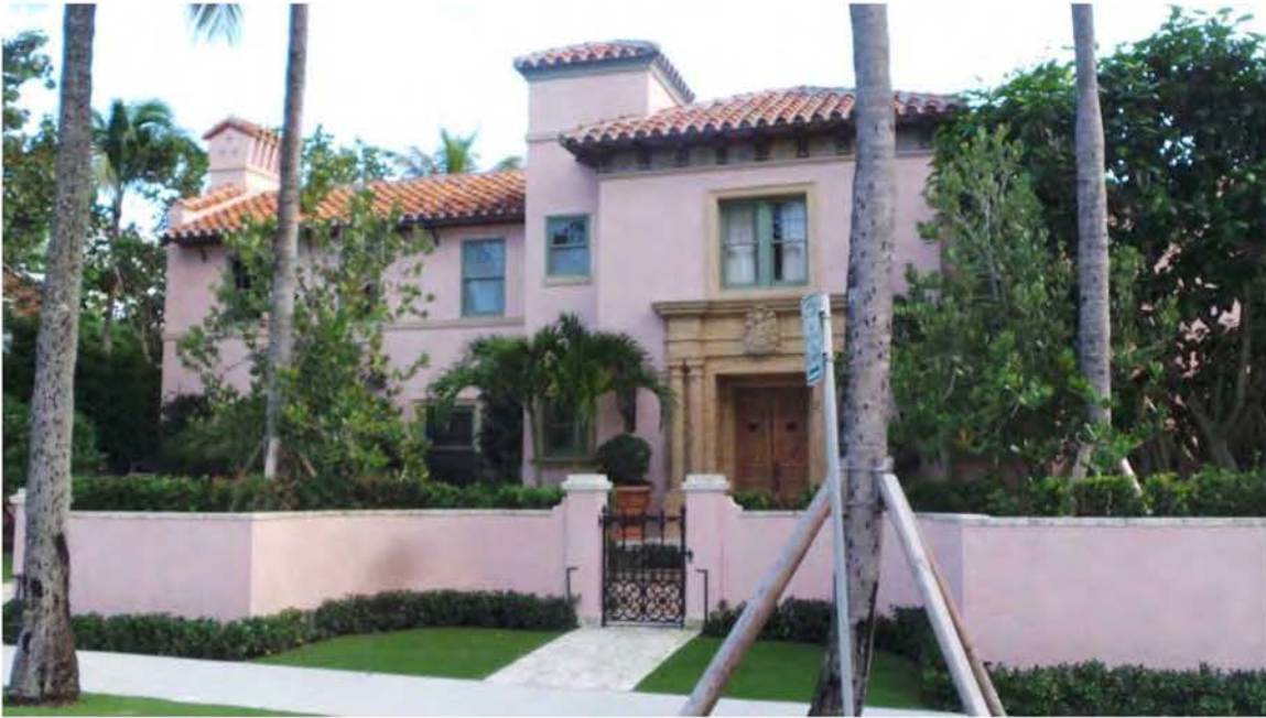
Main (North) Facade
