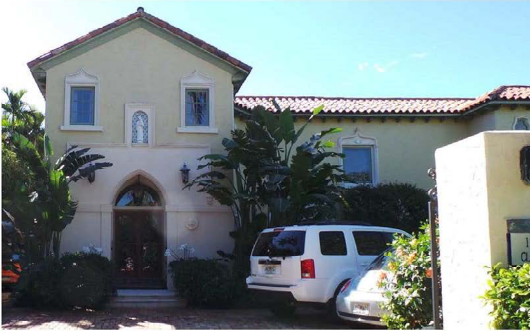
Eastern Wing and Central Bay
