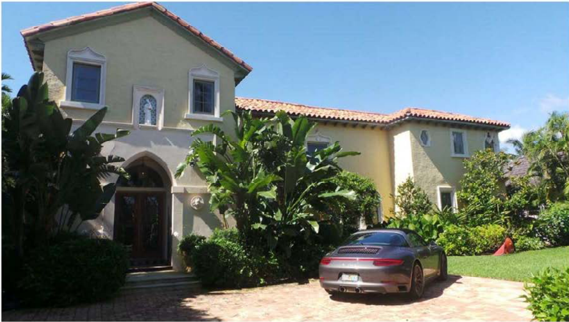
Main (North) Façade
