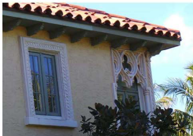
Decorative Tracery at Northwest Corner
