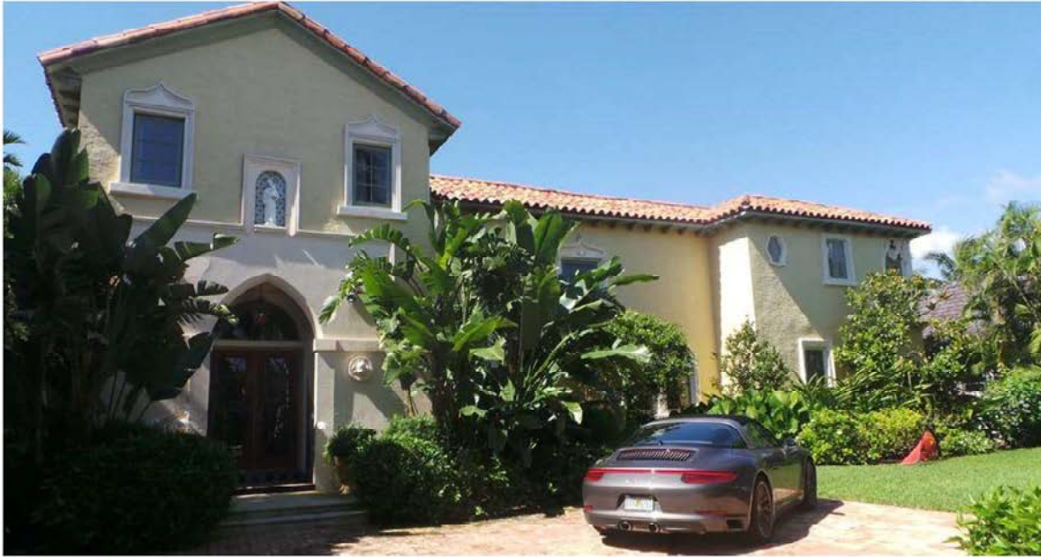
Main (North) Facade
