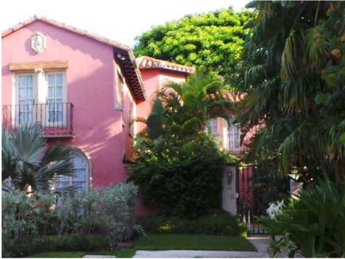
Entrance Courtyard at East End of Property
