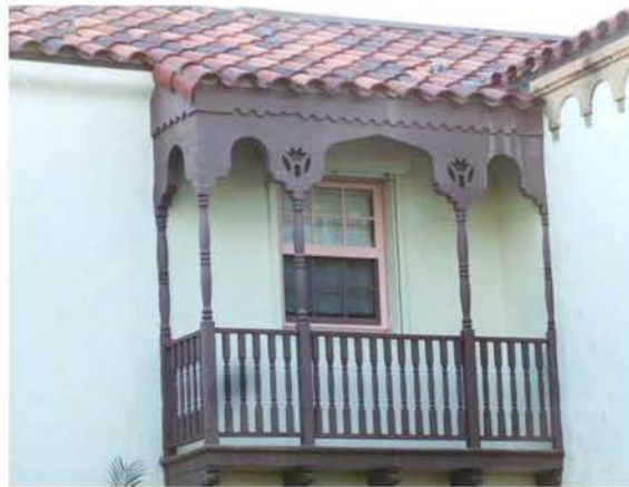
Main Façade Balcony
