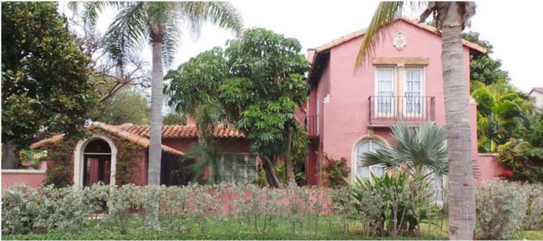
Main (South) Façade
