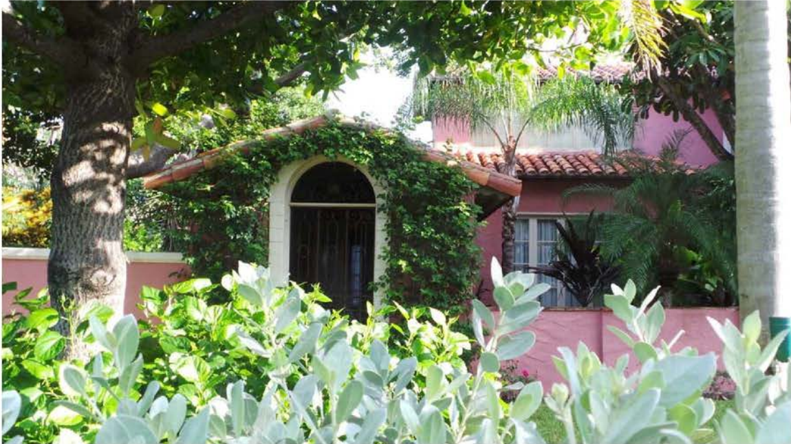
Breezeway – South Facade
