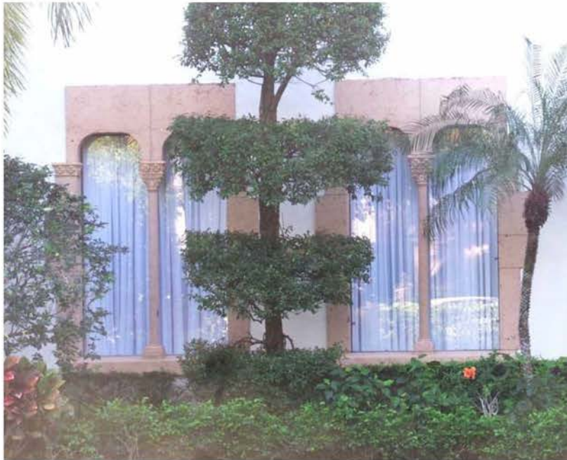
Windows on East End on North Façade
