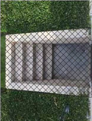
PUMP ROOM STAIR REMOVAL
