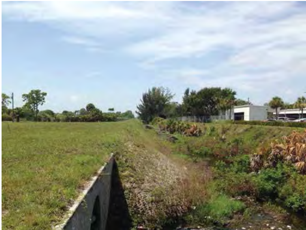
Subject Site on the Left, Looking South at the Drainage Feature along the West Line of the Subject
