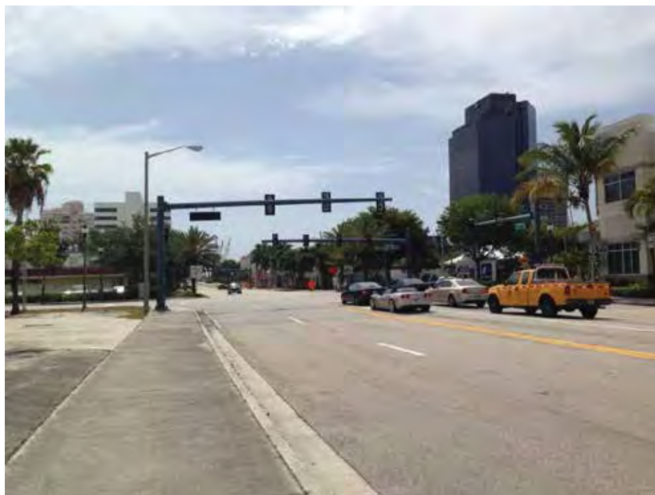
N. Quadrille Boulevard Looking East Toward N. Dixie Highway
