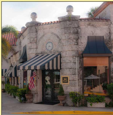
[ chamfered wrap framed with piers ]
