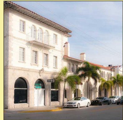
[ taller building anchoring block corner ]
