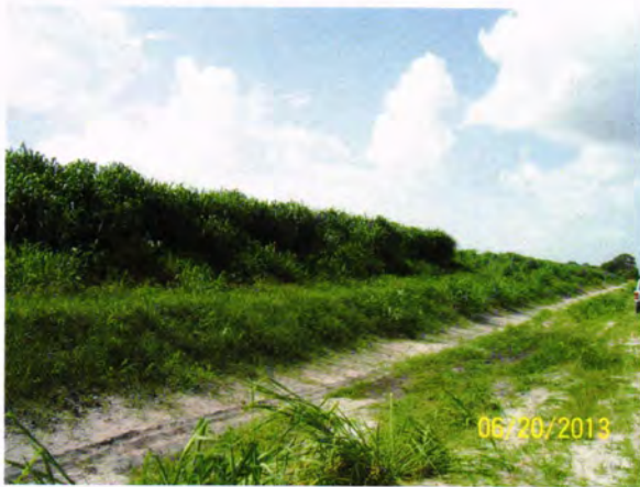
Western side view of the landfill
