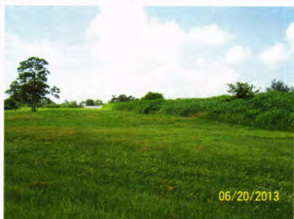
Eastern side view of the landfill
