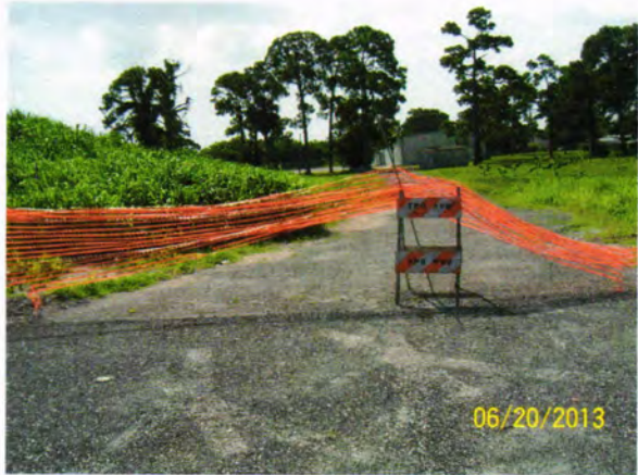
New perimeter road on south side
