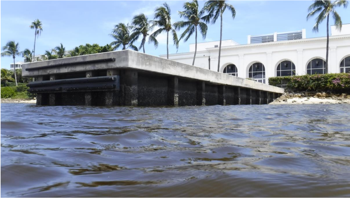
3. Western portion of the property, facing northeast.
