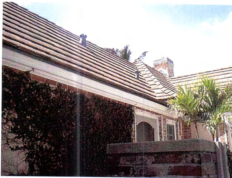
Tie-in of 32.6' Bedroom Wing Addition at Roof Line to Original Home
