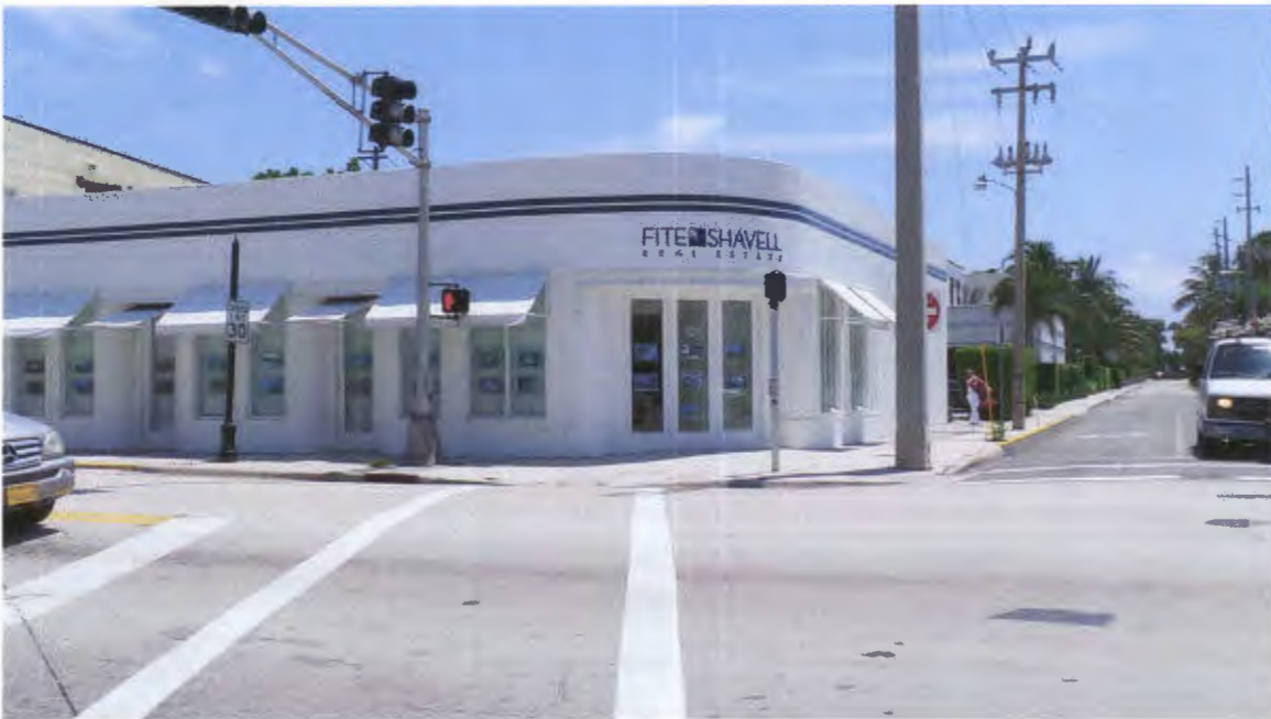
#18. 101 North County Road
