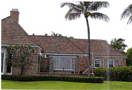
Fig. 9. Dining Room pavilion at center showing bay window covered by storm shutters in place of original pair of double-hung windows, affecting the rhythm and scale of the facade.
