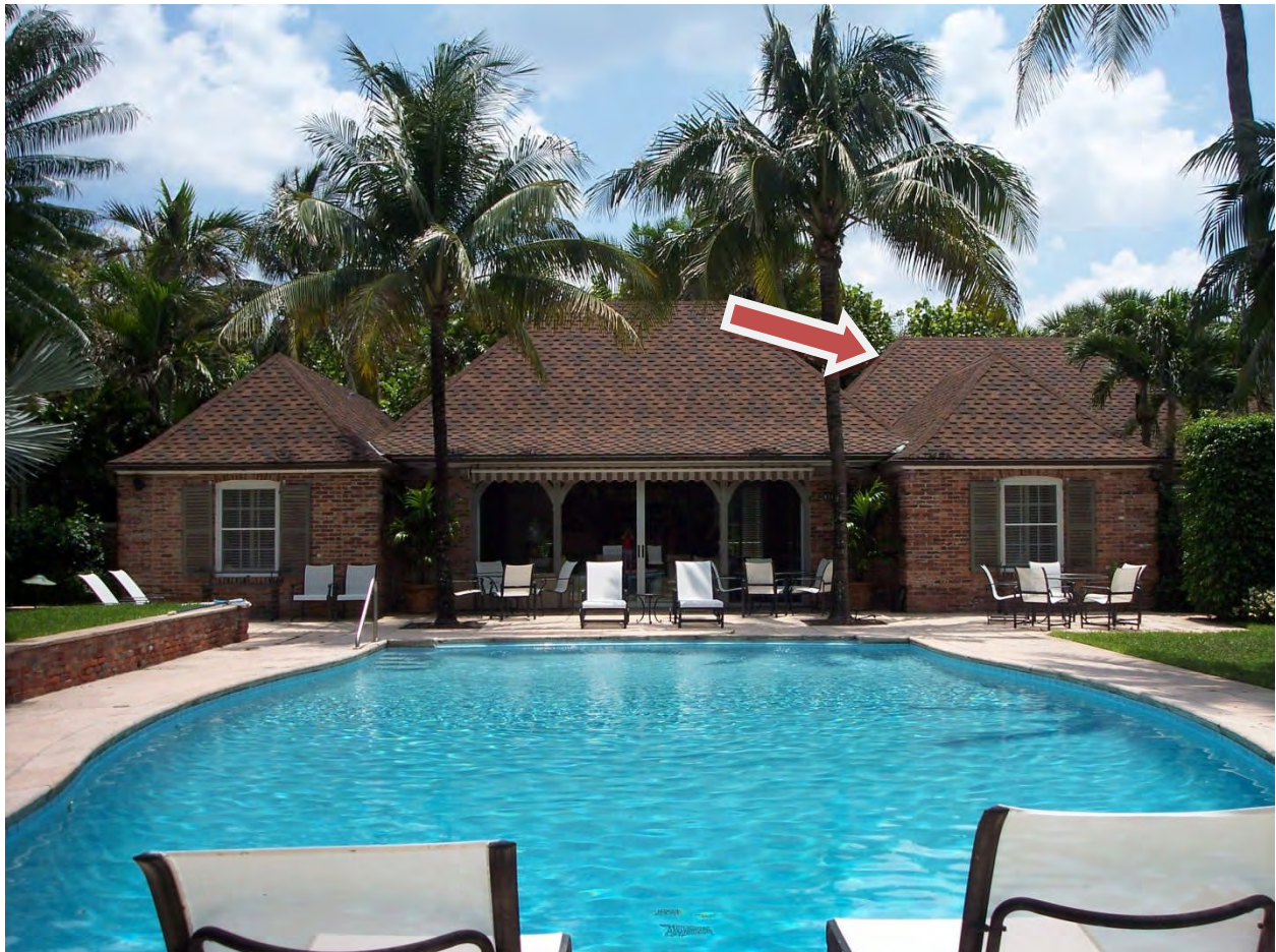
The Guest House Addition is Not Mentioned in the Landmark Report
