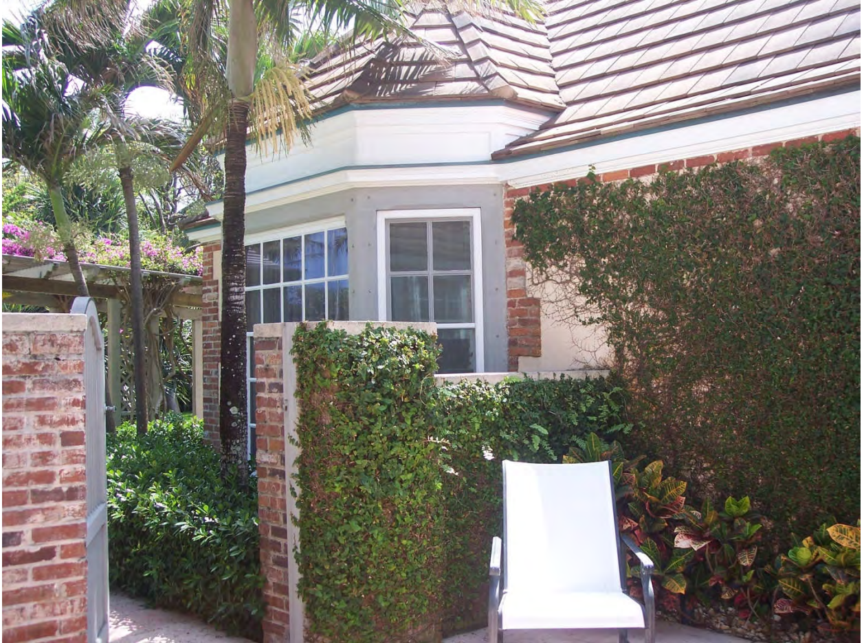
View of the north wall of the southwest bedroom addition to the main house.
