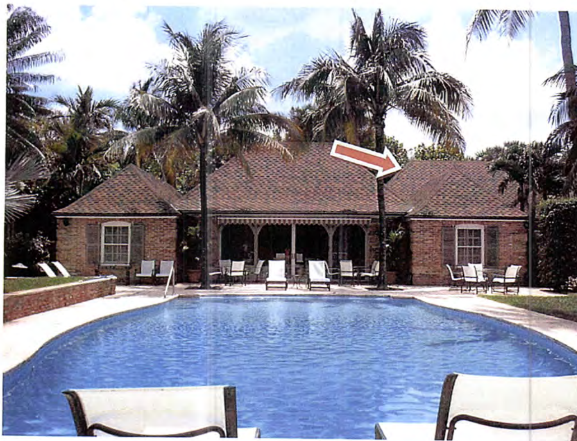
The Guest House Addition is Not Mentioned in the Landmark Report
