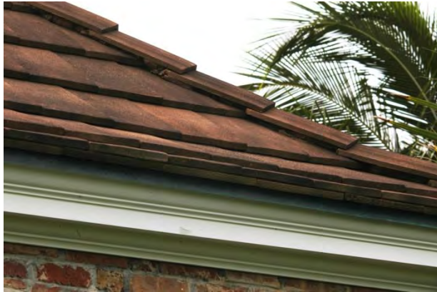
Figs. 12 and 13, New shingles on left (2007) compared with original shingles on the right (1937), which were salvaged and used on the cabana roof.
