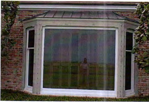
Figs. 14 and 15, Note the roof over the bay window, replaced in copper standing seam (1974), as opposed to the original which was tile. Guest House roofing was changed from shake shingle to GAF or composition shingles in 2003.
