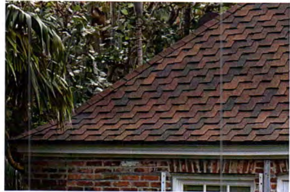
Figs. 14 and 15, Note the roof over the bay window, replaced in copper standing seam (1974), as opposed to the original which was tile. Guest House roofing was changed from shake shingle to GAF or composition shingles in 2003.
