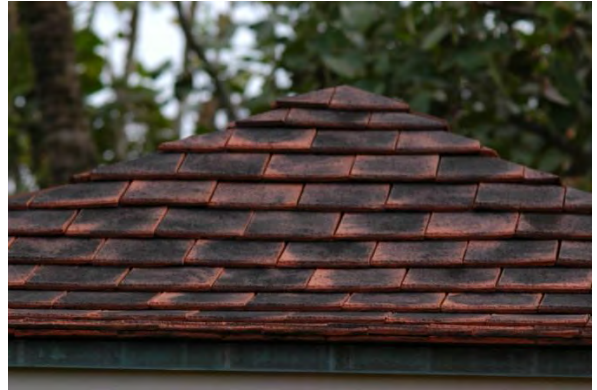
Figs. 12 and 13, New shingles on left (2007) compared with original shingles on the right (1937), which were salvaged and used on the cabana roof.
