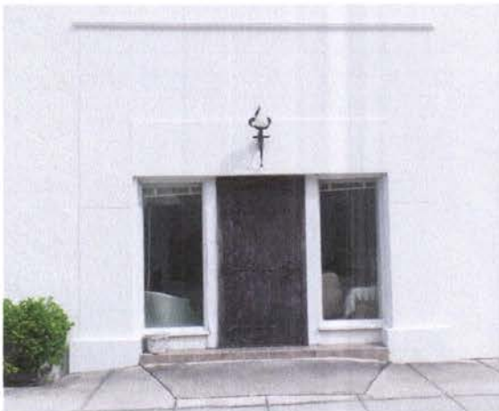
Entrance on South Facade
