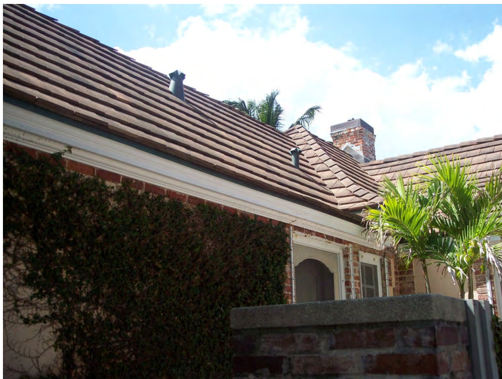
Tie-in of 32.6' Bedroom Wing Addition at Roof Line to Original Home
