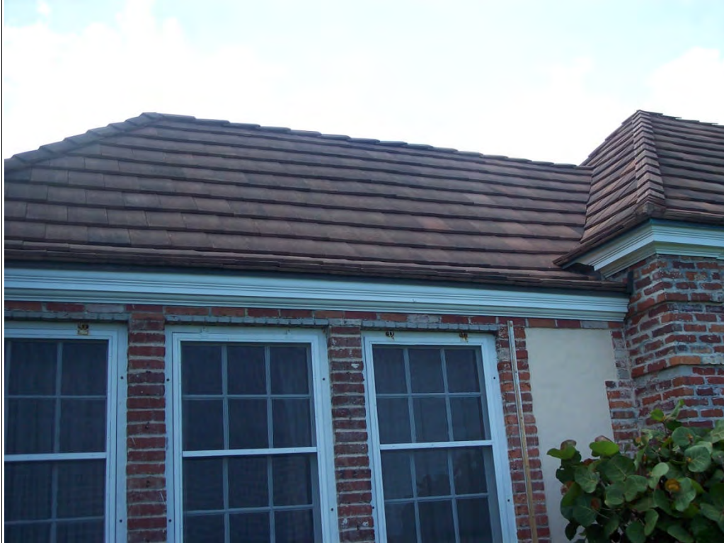
Tie- in at Roof Line from Sitting Room to Original Portion of Home
