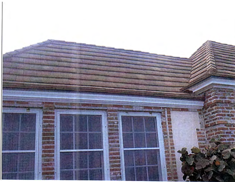
Tie- in at Roof Line from Sitting Room to Original Portion of Home
