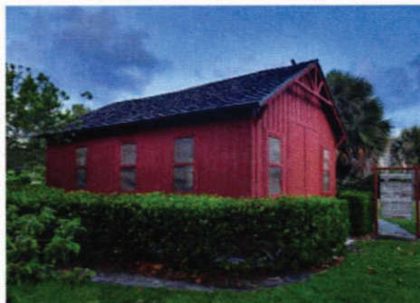
3 CORNER VIEW OF WEST & NORTH SIDES
