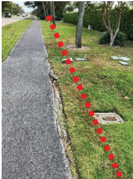
Existing Water Meter and Irrigation Valve Boxes
