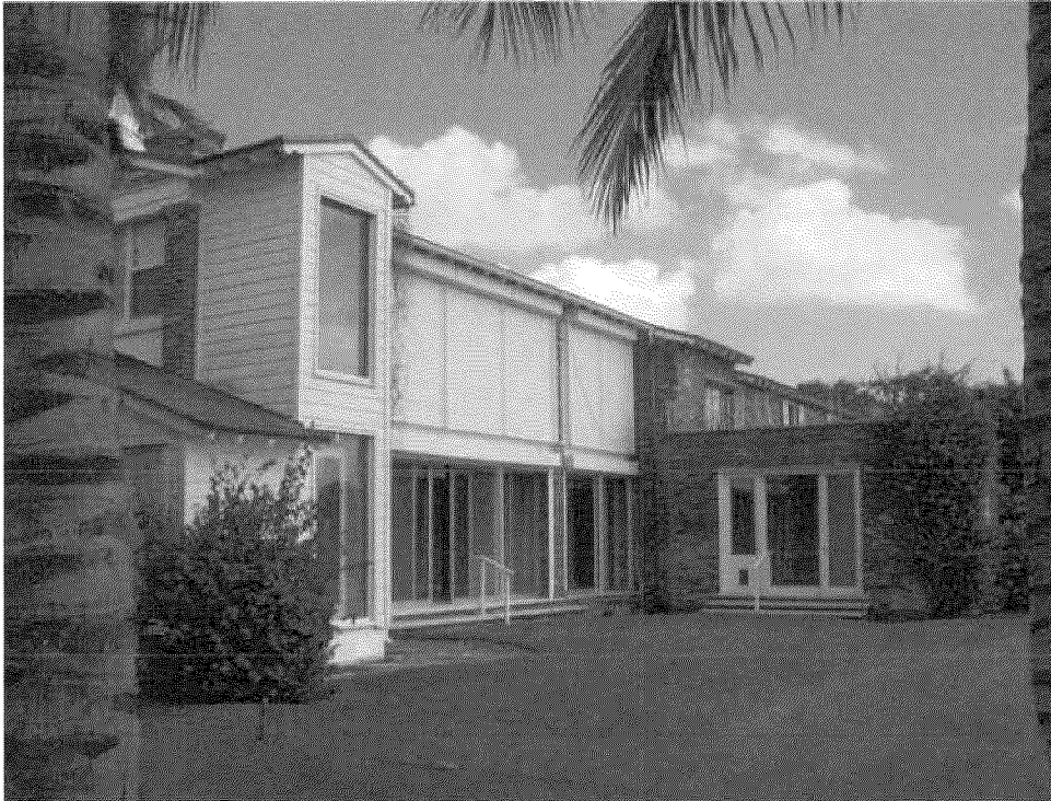
Existing conditions on the south facade showing elevator and dining room which will be removed in the present restoration.
