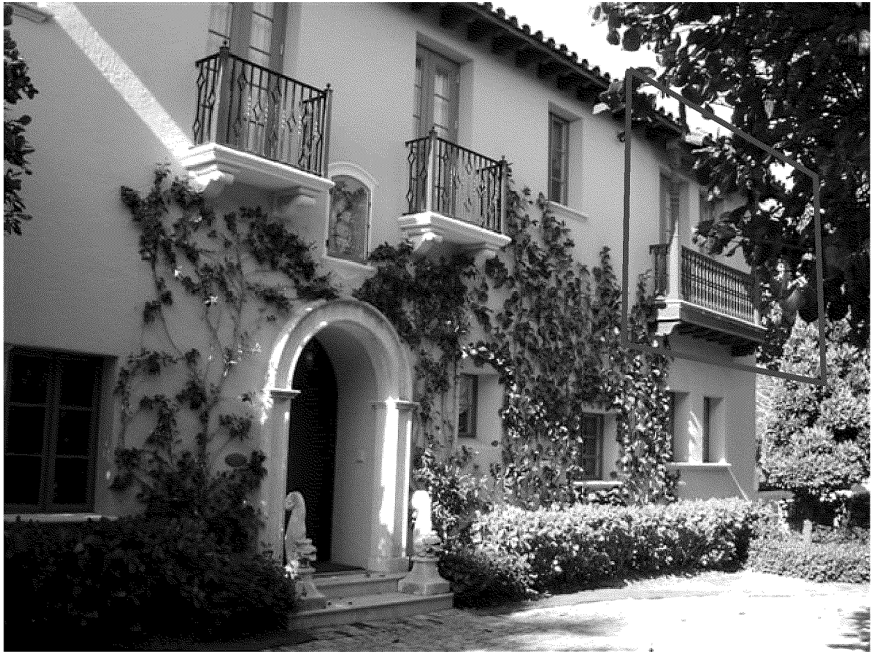
Fig. 13 View of the North façade, showing the altered wall in red outline. The raised wall in this area permitted the construction of an additional guest bedroom. The wooden balcony was also created to complement those on the east façade. Photo by James Norquest, 2011.
