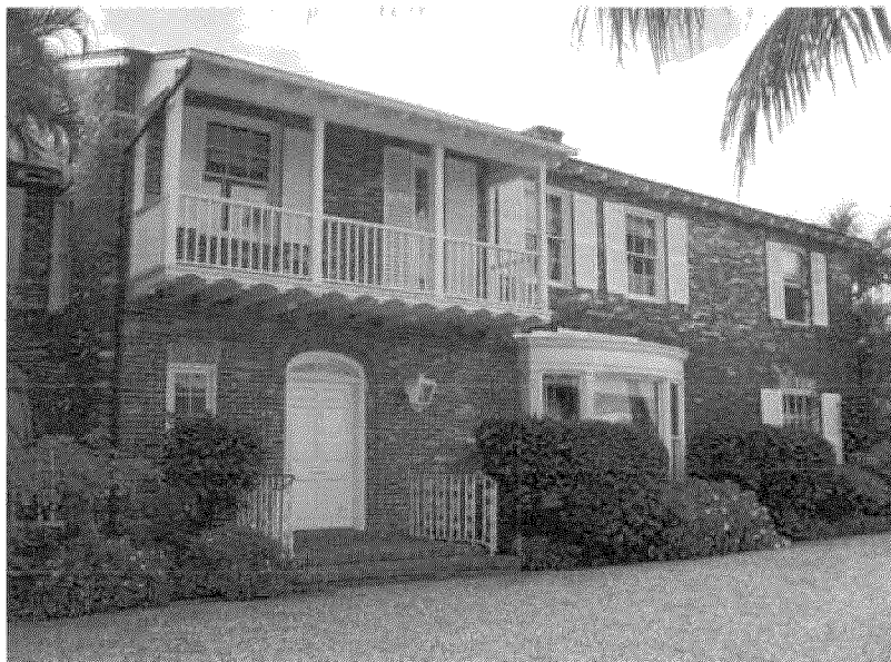
The front (north) facade showing entry and cantilevered balcony
