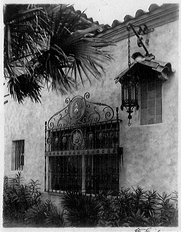
Fig. 5 Detail of North Façade showing ornamental wrought iron grille, lantern and pent roof, none of which presently exists. The lost iron work was custom-made to the architect's specifications and probably produced by the Los Manos factory, founded by Mizner. Photograph by Frank E. Geisler, Preservation Foundation of Palm Beach.
