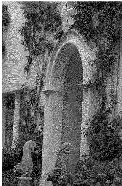
Figs. 16 and 17 Detail views of the north façade showing the raised portion of the wall in the second story and the portal surround. Neither of these features are historic. The new balcony does not match those on the east facade which are less tall or attenuated in comparison.
