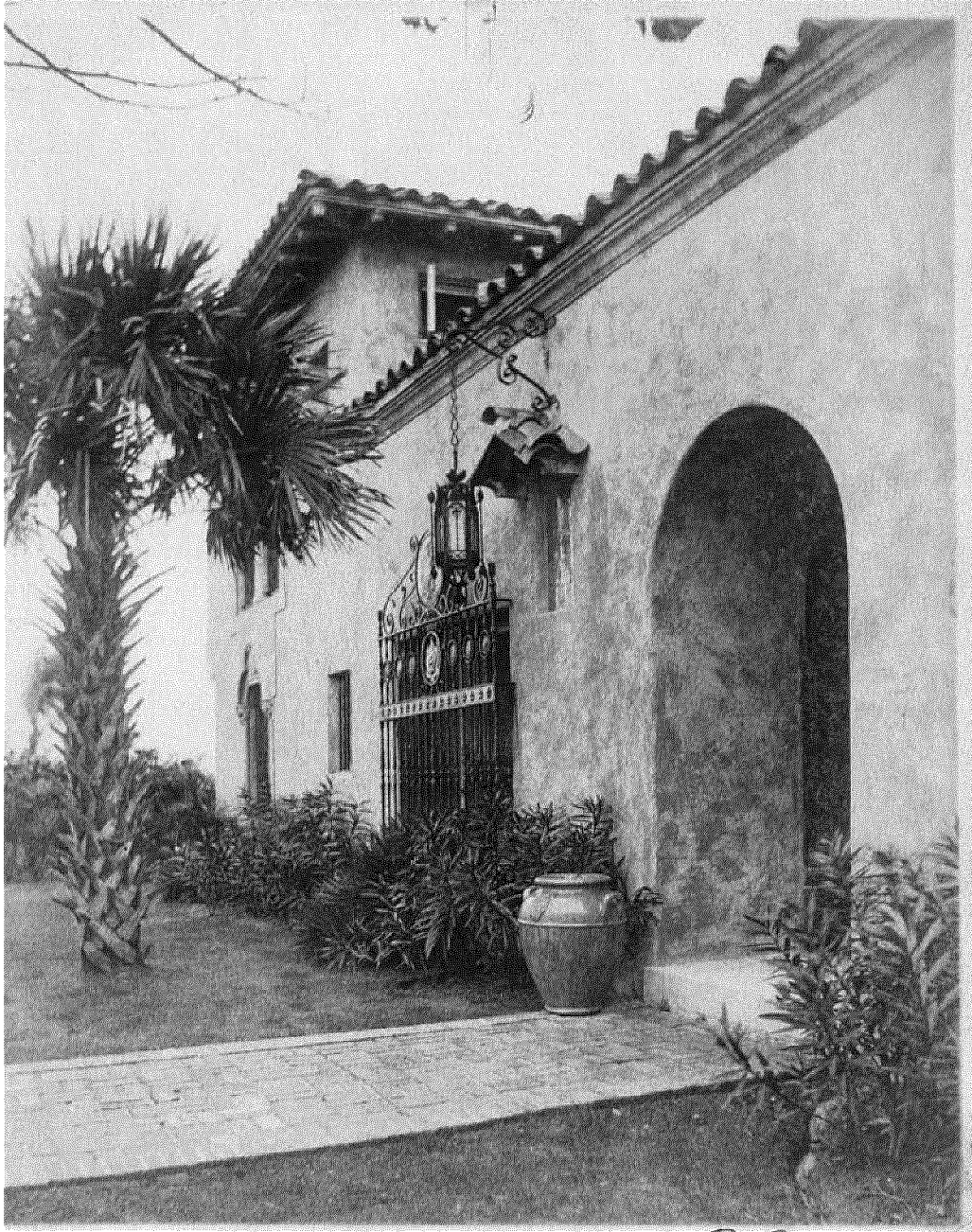
Fig. 4 North Façade from entry portal looking southeast. Note the single- story entry bay. In a departure from the architect's drawings, there is no ornamental treatment of the portal, no rusticated stone or stucco surround. As shown, the only rooms to occupy the second story are the master bedroom and bath. The present façade bears no resemblance to the original. Photograph by Frank E. Geisler, Preservation Foundation of Palm Beach.
