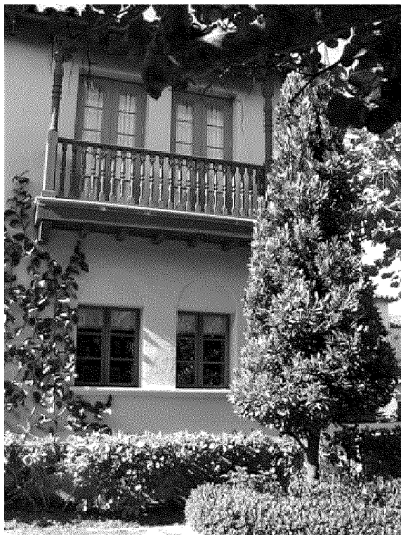
Figs. 16 and 17 Detail views of the north façade showing the raised portion of the wall in the second story and the portal surround. Neither of these features are historic. The new balcony does not match those on the east facade which are less tall or attenuated in comparison.
