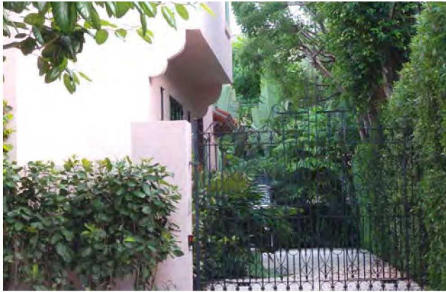
Portion of West Façade
