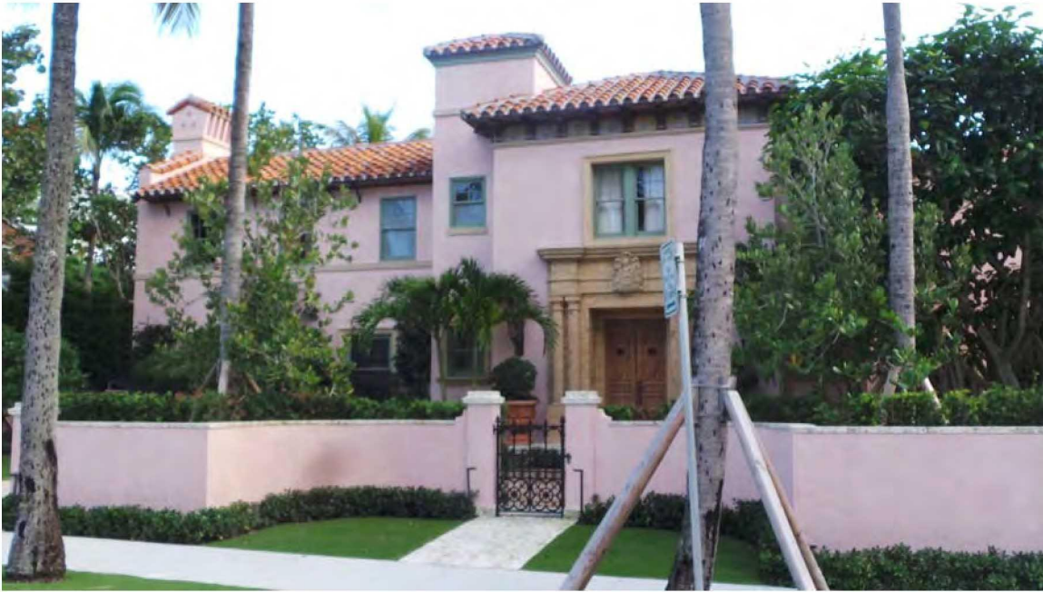
Main (North) Facade
