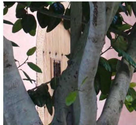
Door on West Façade
