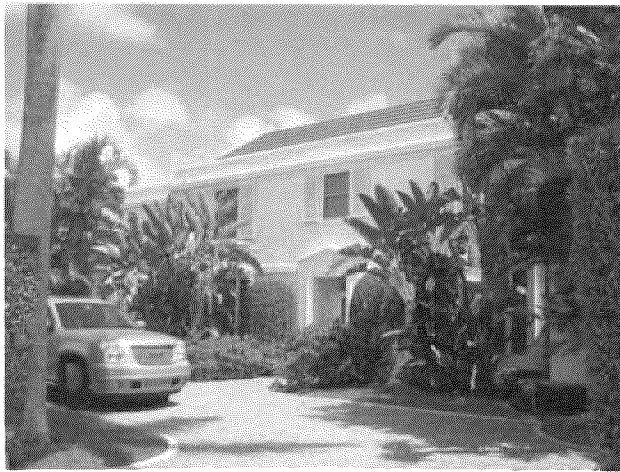
235 Sanford Avenue, Wyeth and King, 1940
