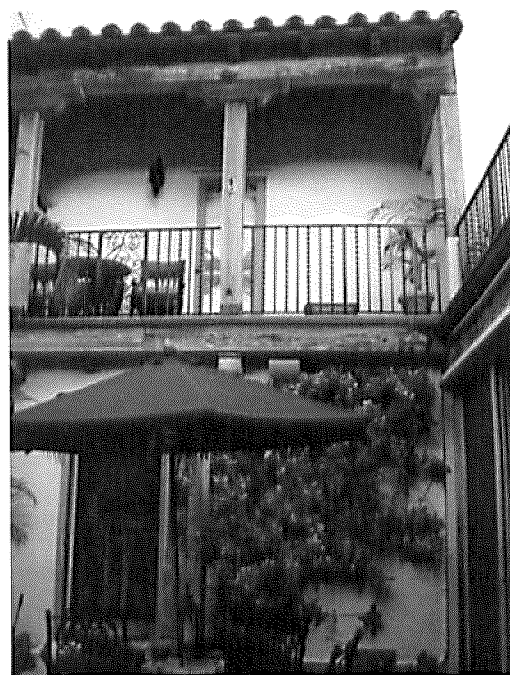
The second floor rear balcony
