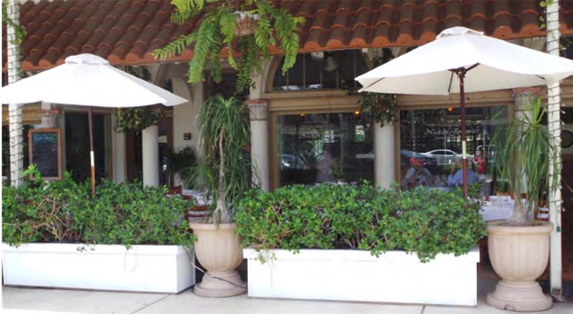
207 Royal Poinciana Way – South Façade Colonnade
