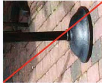
FIGURE 5 Domed stanchion bases are not permitted
