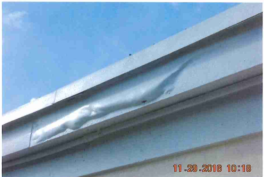
#2 Example of water blister in paint at fascia, east side, typical of 2.
