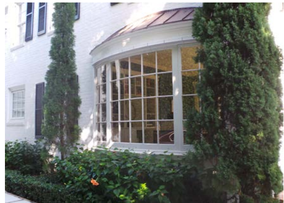
Bow Window on West Facade
