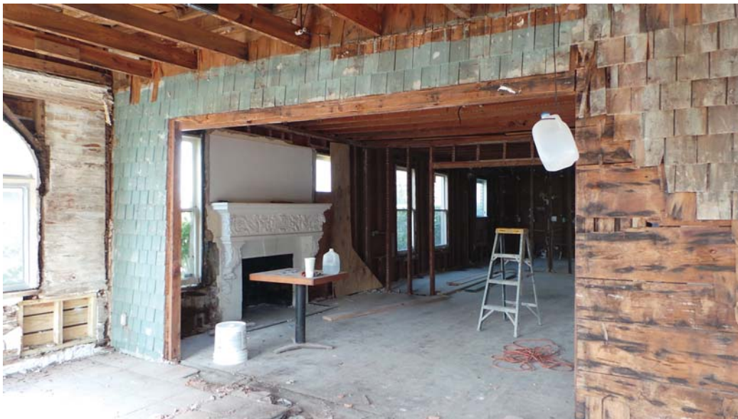
Shingle Siding from Original Design and Fireplace Mantel
