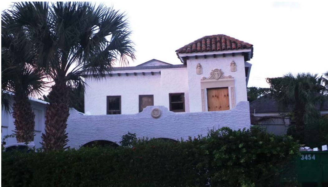
Main Façade Showing Gable Roof Over Fan
