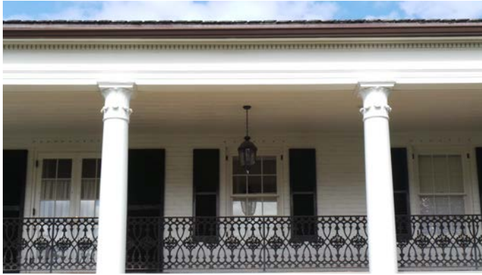
Detail of Porch Columns, Entablature & Railing
