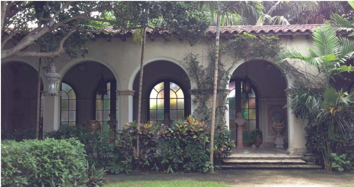
Loggia, Looking South From Courtyard
