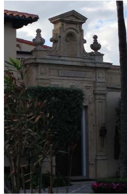
East Façade - Entrance
