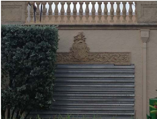
East Façade – Decorative Lintel Over Window
