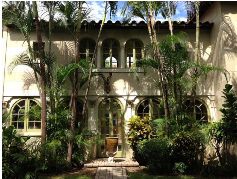
South Façade, Showing First and Second Story Additions
