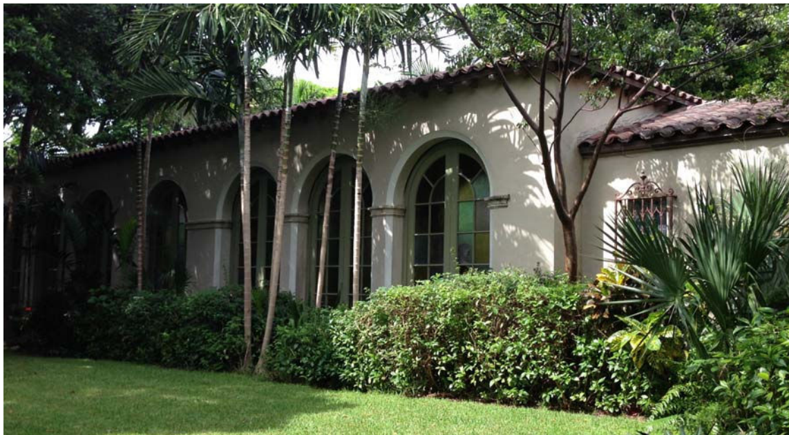
South Facade of Loggia Addition with Ironwork Removed
