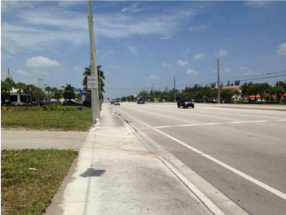
Okeechobee Boulevard Looking West from the Subject
