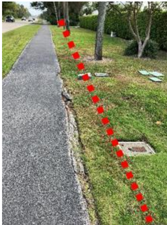
Existing Water Meter and Irrigation Valve Boxes
