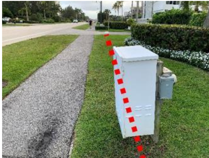
Existing Communications Utility Panel
