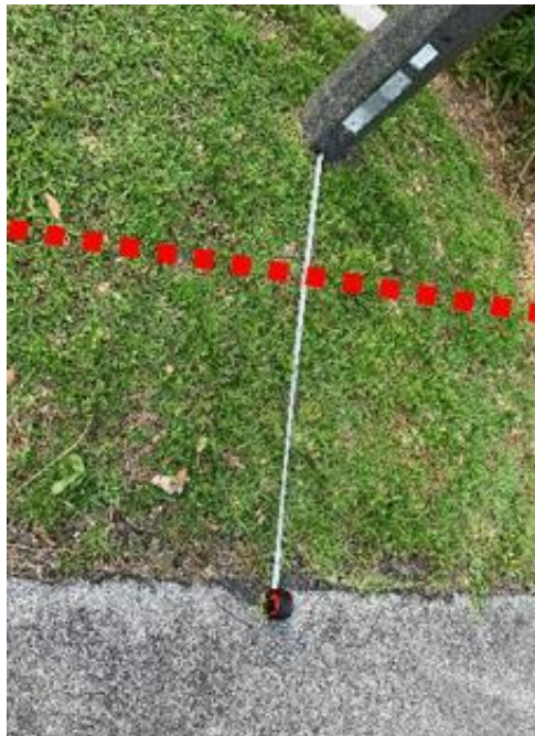
Existing Street Lighting Pole
