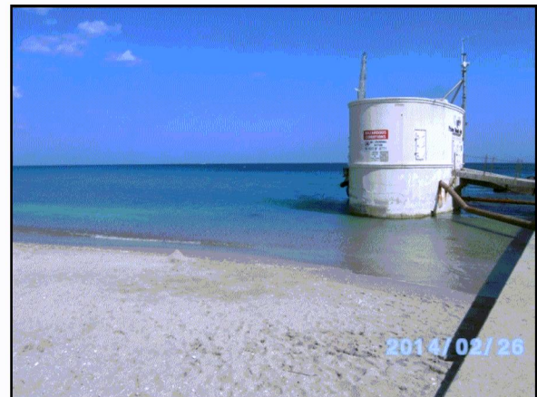
Sand Transfer Plant at the Lake Worth Inlet's north jetty.
