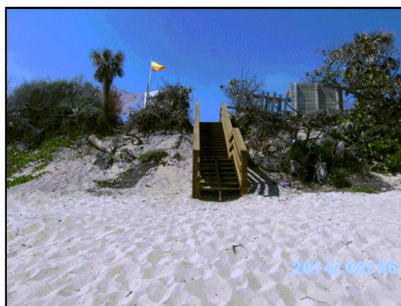
New access point staircase at the south end of Phipps Ocean Park.
