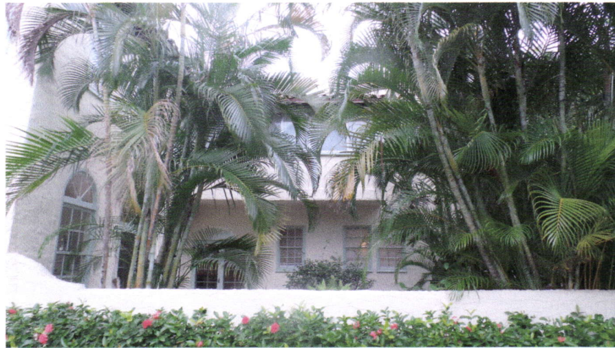
East Façade with Second Story Porch
