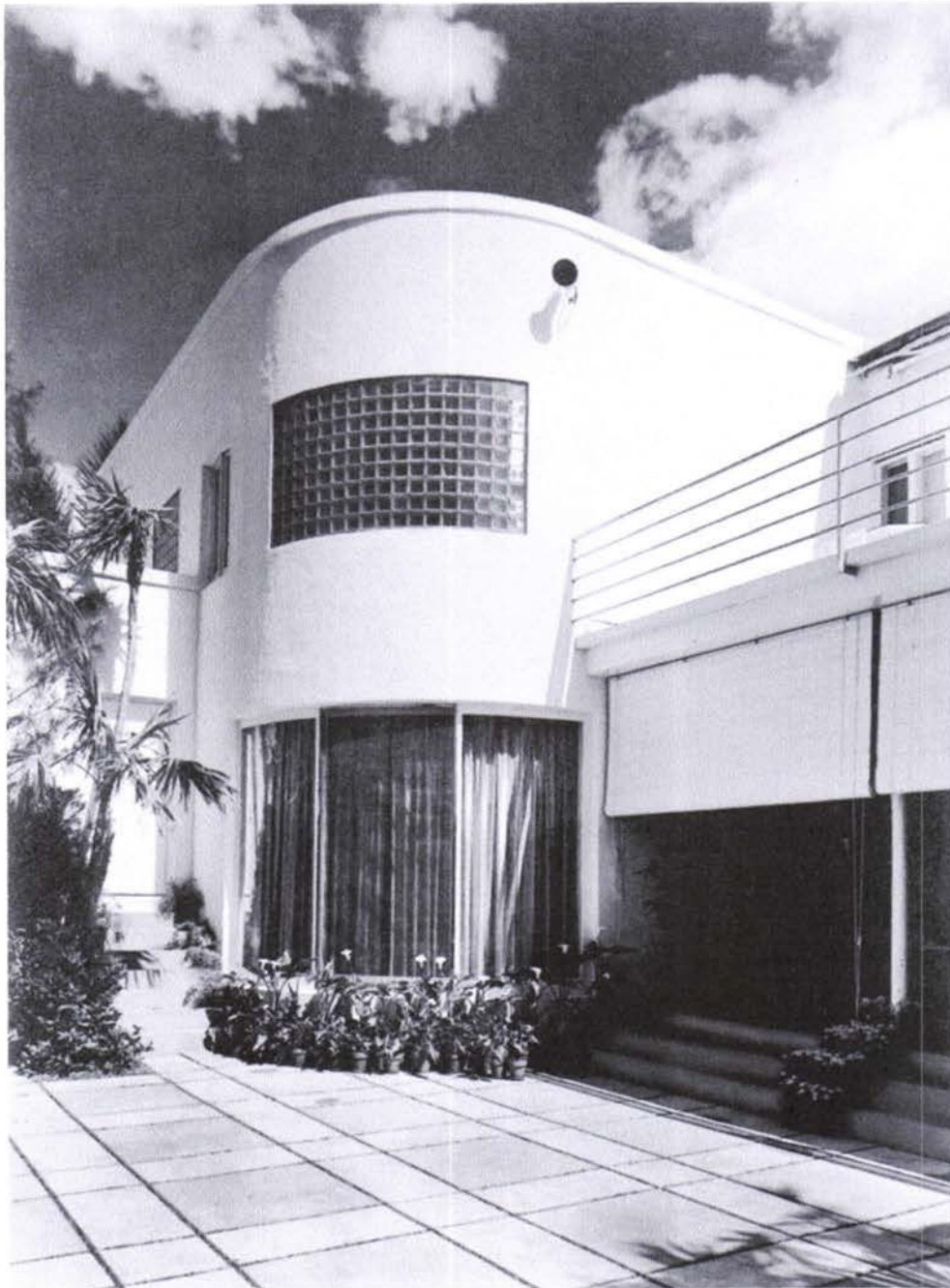
Curved Wall Containing Glass Blocks Courtesy of the John L. Volk Foundation
