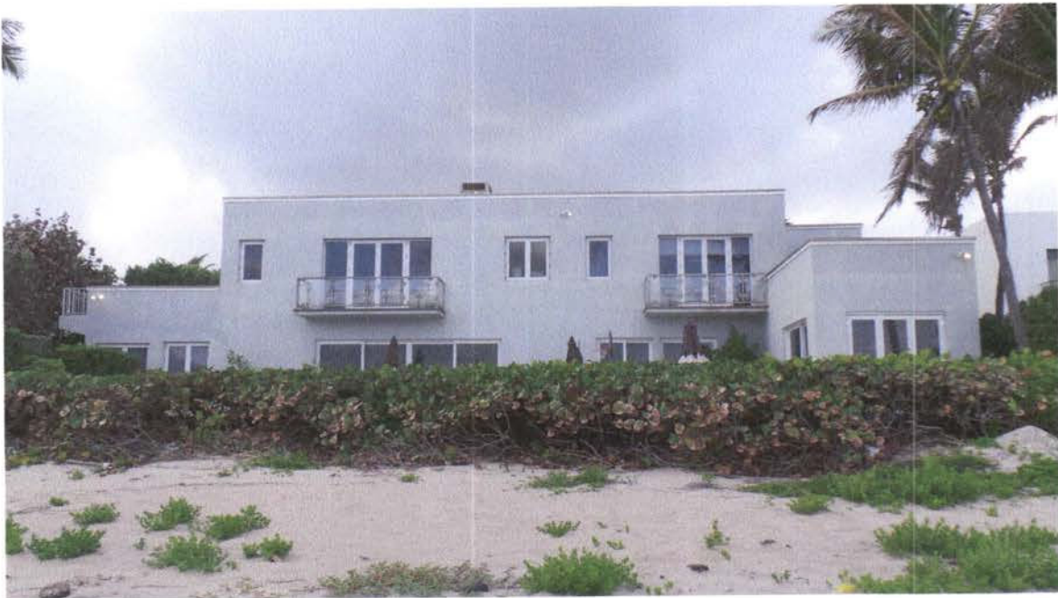
Rear (East) Facade
