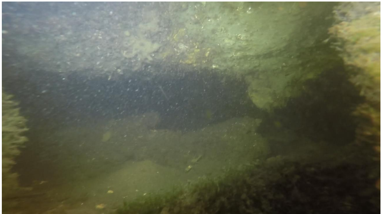
Figure 3.12: Sta 15+15. Gap underneath the corrugated section of the bulkhead and vague outline of a secondary sheet pile wall in the background.
