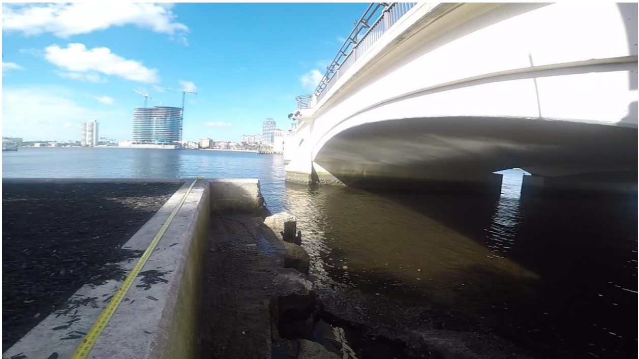
Figure 3.8: Sta 0+02 looking west. Corrugated face and offset cap.
