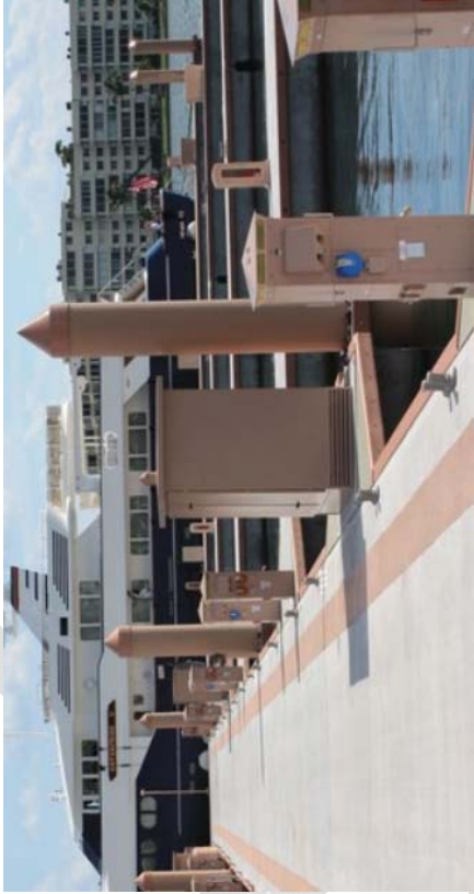
Figure 6.1: Typical Pedestal for Electrical, Water and Internet/Phone connection (Palm Harbor)
