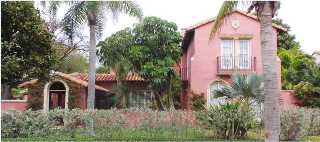
Main (South) Façade
