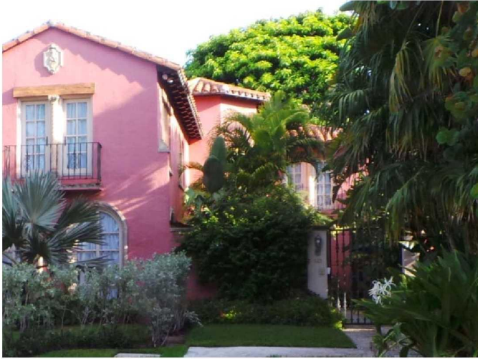
Entrance Courtyard at East End of Property
