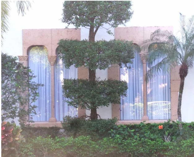
Windows on East End on North Façade
