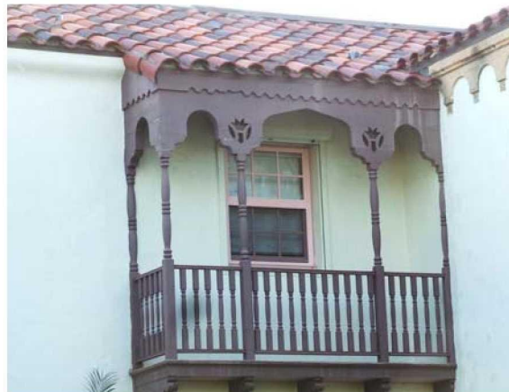
Main Façade Balcony
