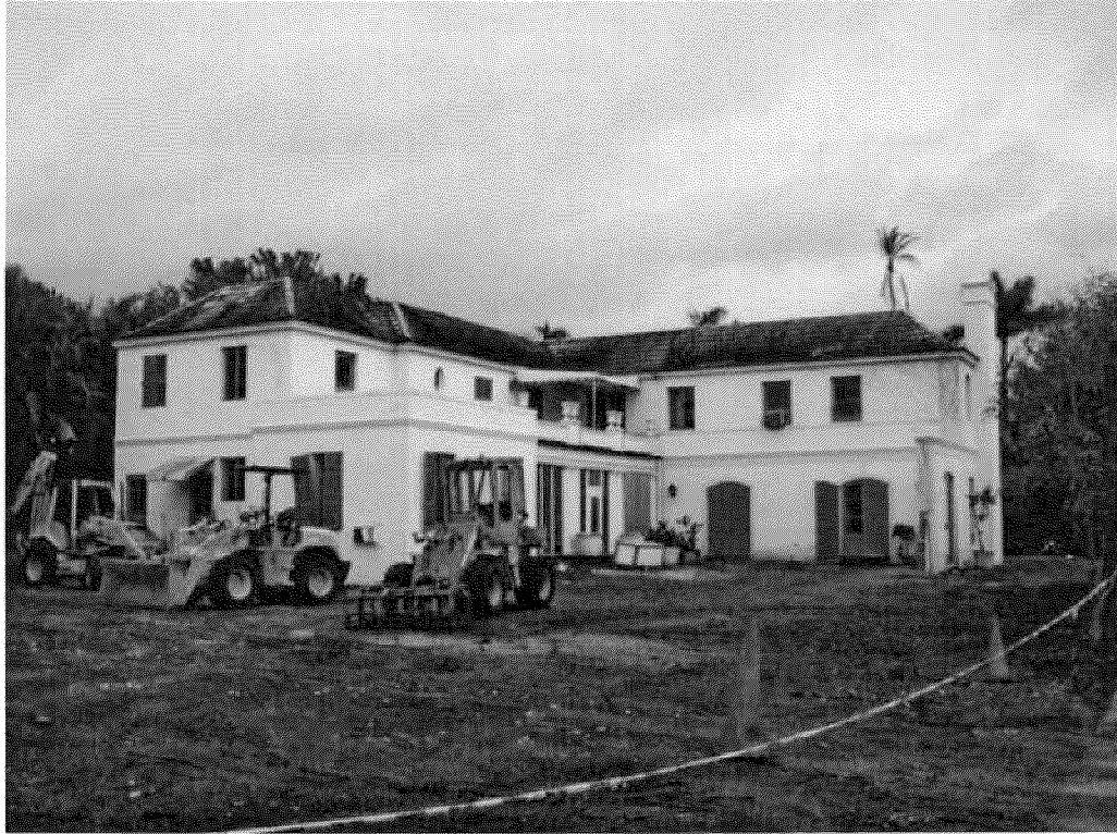
The rear of 300 Barton including the southwest wing of the house.
