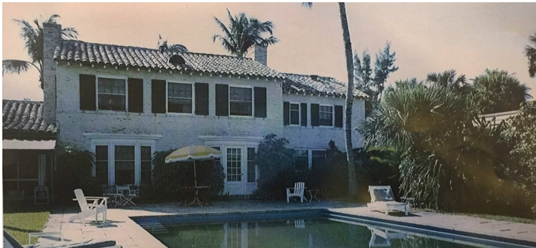
Rear Façade - 1936 Photograph Provided by Property Owner
