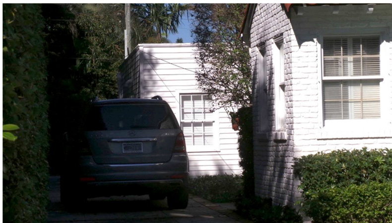
Garage, Looking Northeast
