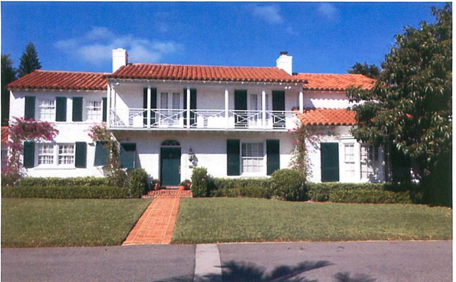
2015 Front View (with 1949 addition)
