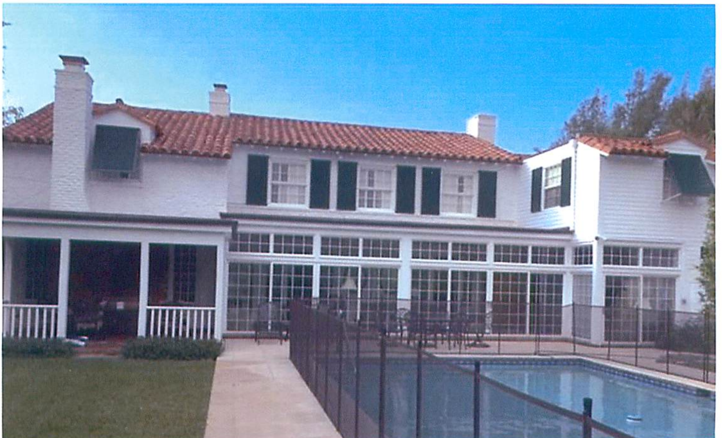
2015 Rear View (with 1949 and 1984 additions)
