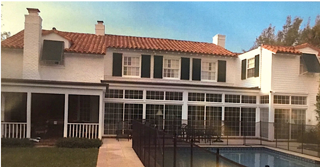
Current Rear Facade Provided by Property Owner
