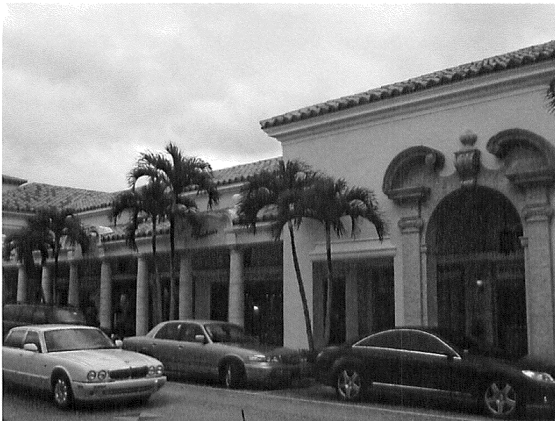
A variety of details help the building read as separate shops. The roof ties the design together.
