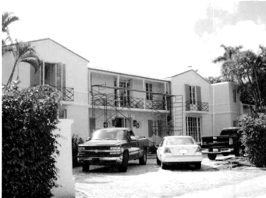
Renovations taking place in 2012.
