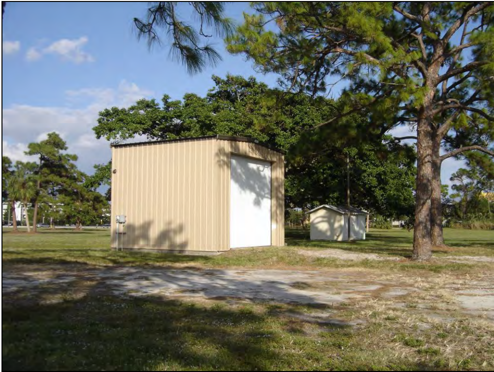
VIEW OF MISCELLANEOUS IMPROVEMENTS
