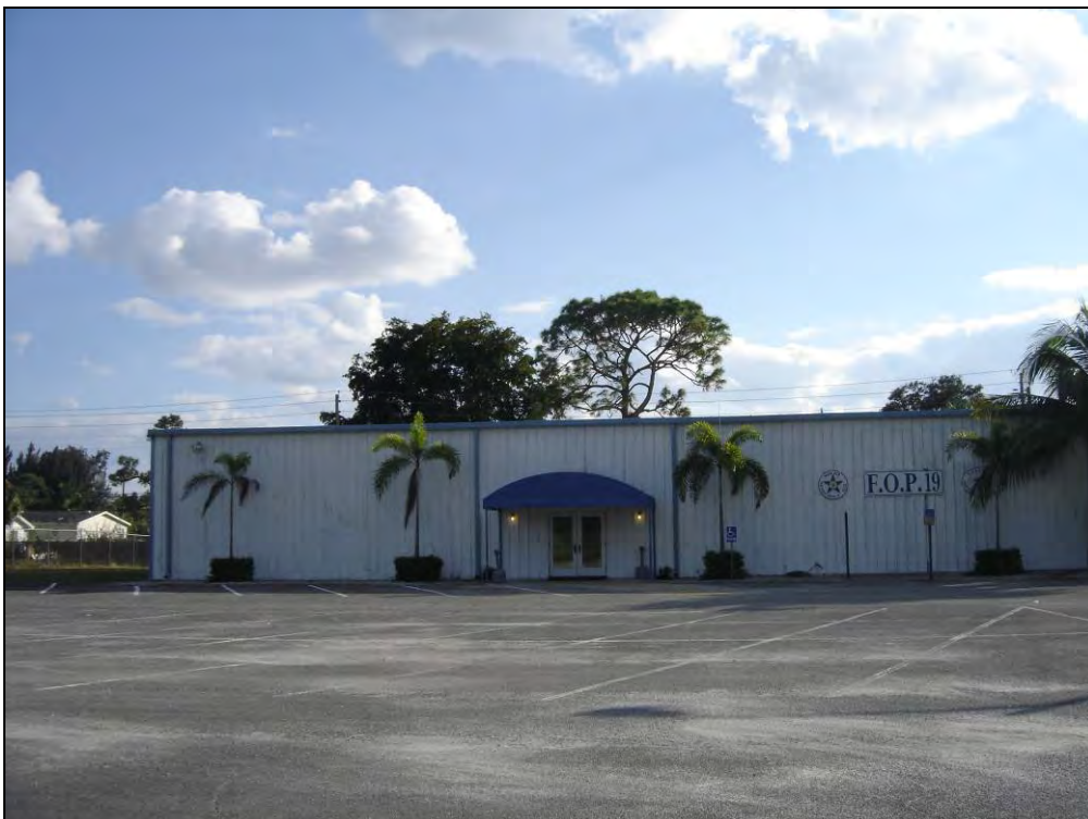
VIEW OF POLICE LODGE BUILDING
