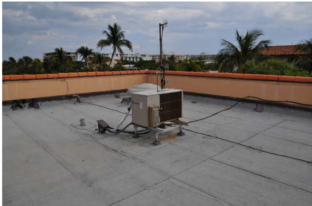
Photograph 12: View of the Liebert system condensing unit.
