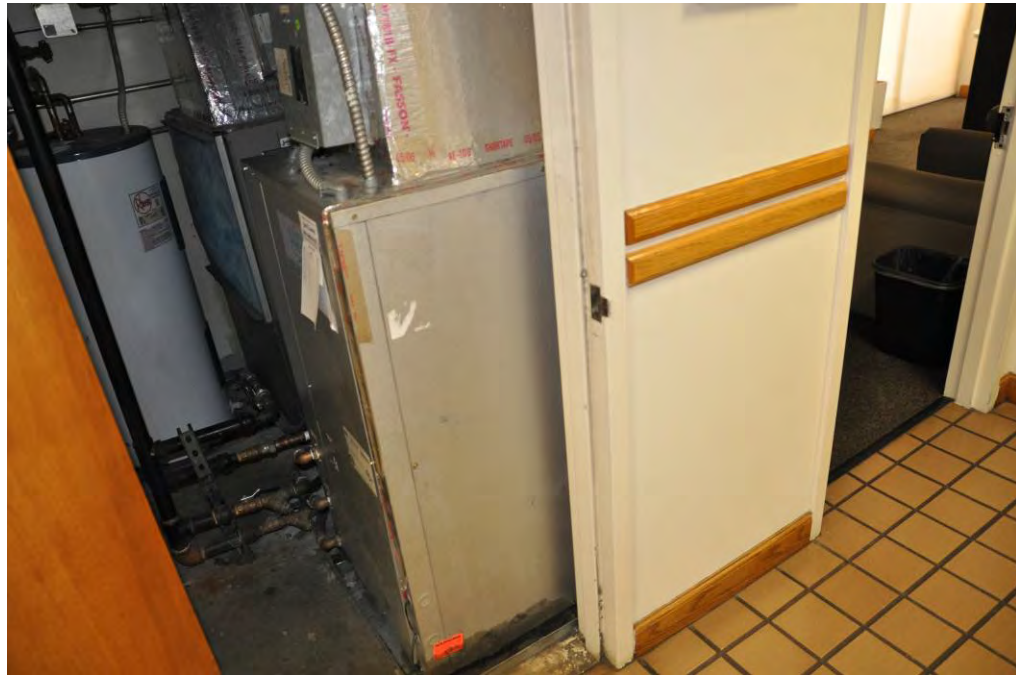
Photograph 8: View of a heat pump located in a mechanical closet.
