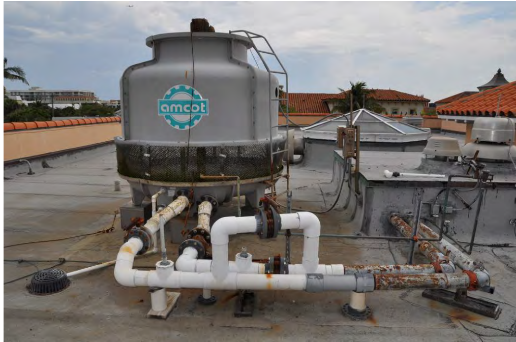
Photograph 4: View of roof mounted condenser water piping.
