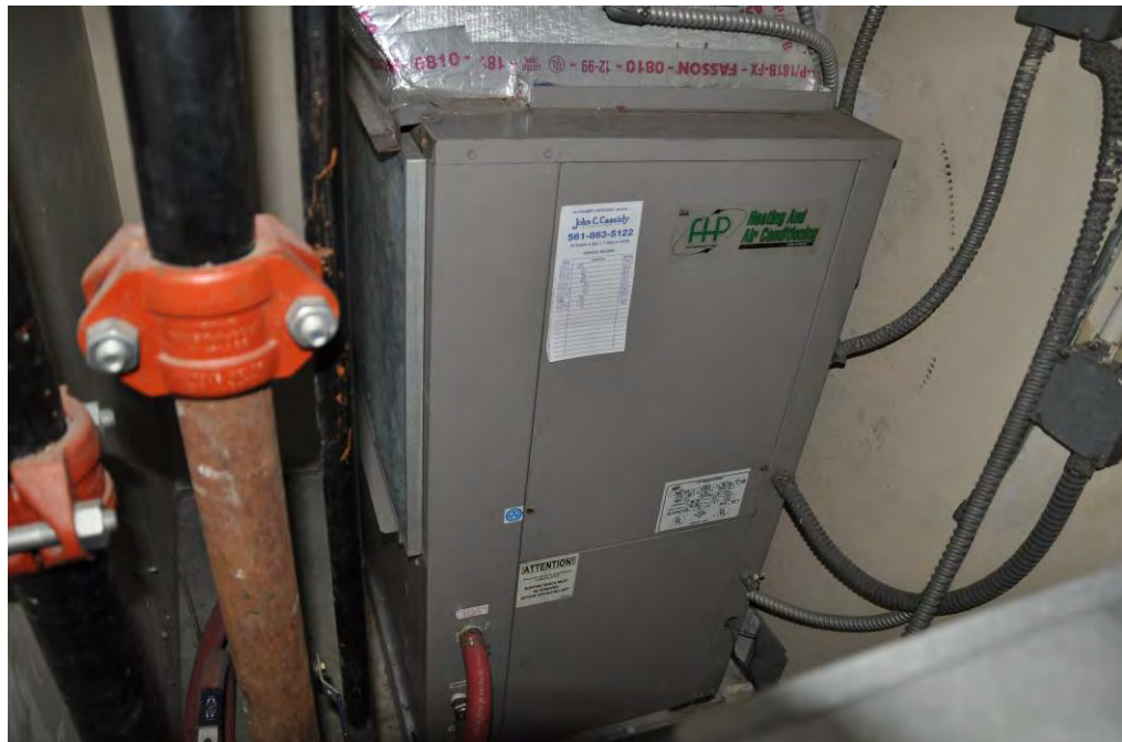
Photograph 8: View of a heat pump located in a mechanical closet.
