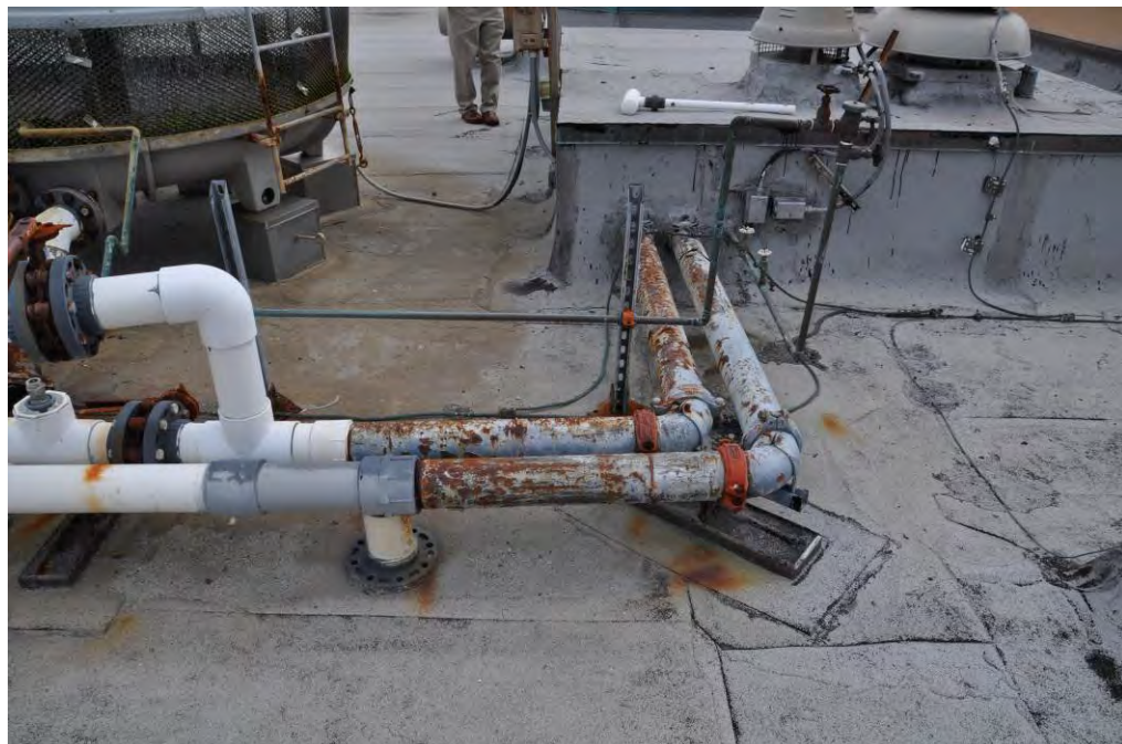
Photograph 4: View of roof mounted condenser water piping.
