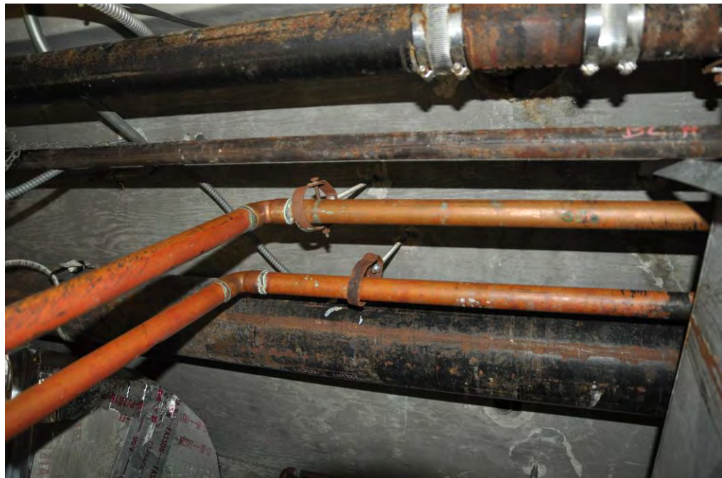
Photograph 6: View of condenser water piping.
