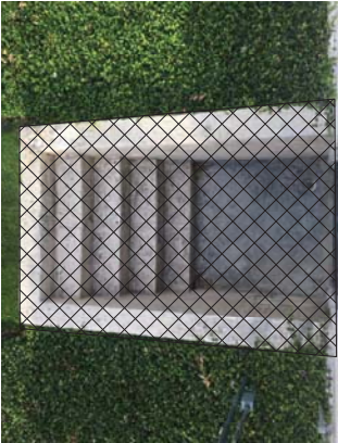
PUMP ROOM STAIR REMOVAL
