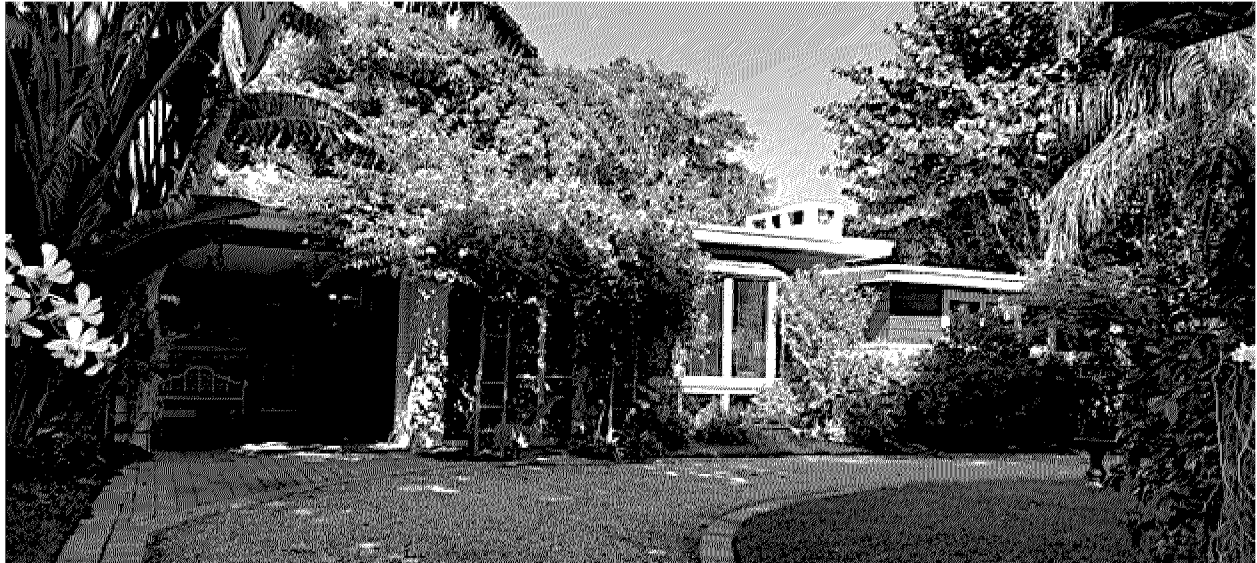
South Façade, Looking Northeast
