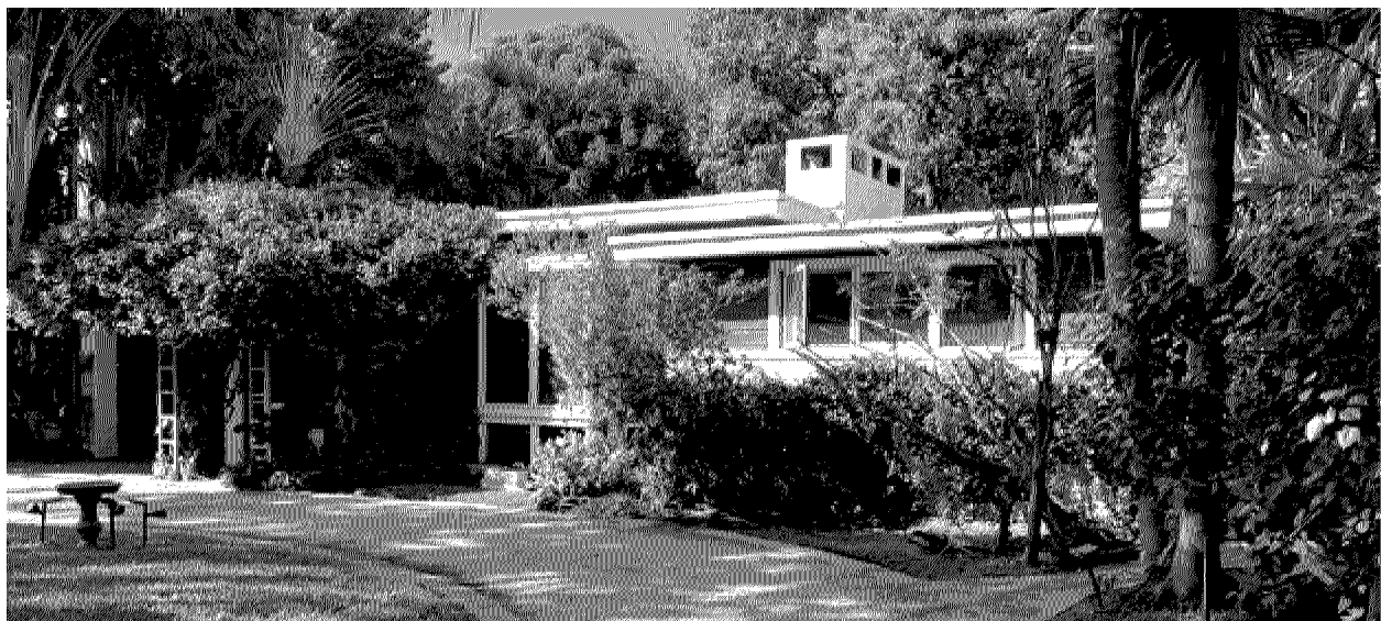
South Façade, Looking Northwest
