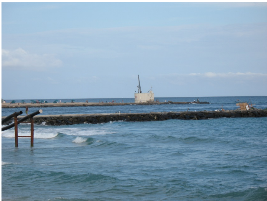
Figure 2. STP discharge pipes (bottom left) in perspective to Lake Worth Inlet jetties and intake facility (middle in distance).
